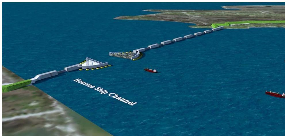
Figure 9: Bolivar Roads Floating Sector Gate with Vertical Lift Gates
