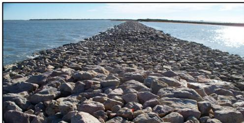
**Erosion Protection of Pelican Island in Corpus Christi Bay** – The project created 1,074 linear feet of additional breakwater (Phase 2), which resulted in a total structure length of 2,384 linear feet (Phase 1 and Phase 2) of a hard substrate that provides aquatic habitat that should benefit fisheries and wildlife resources.
