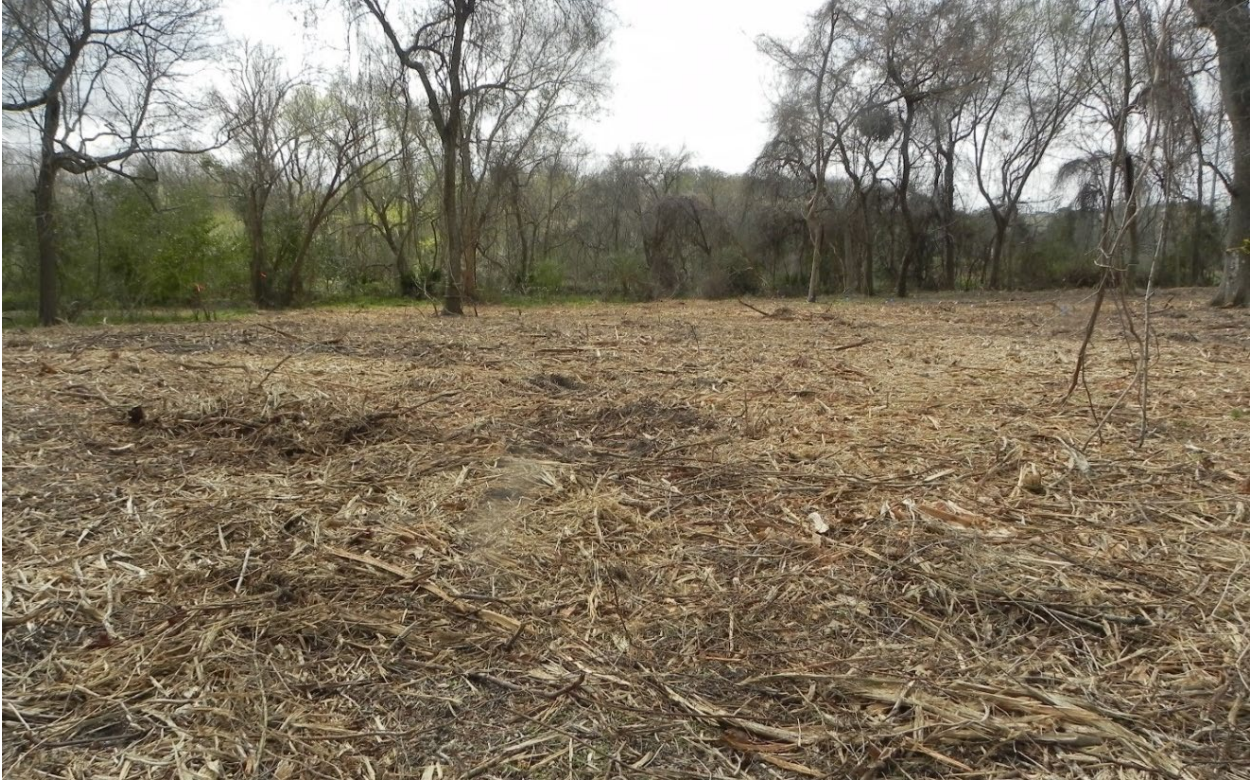
Figure 16. Site After Tree Removal and Mulching
