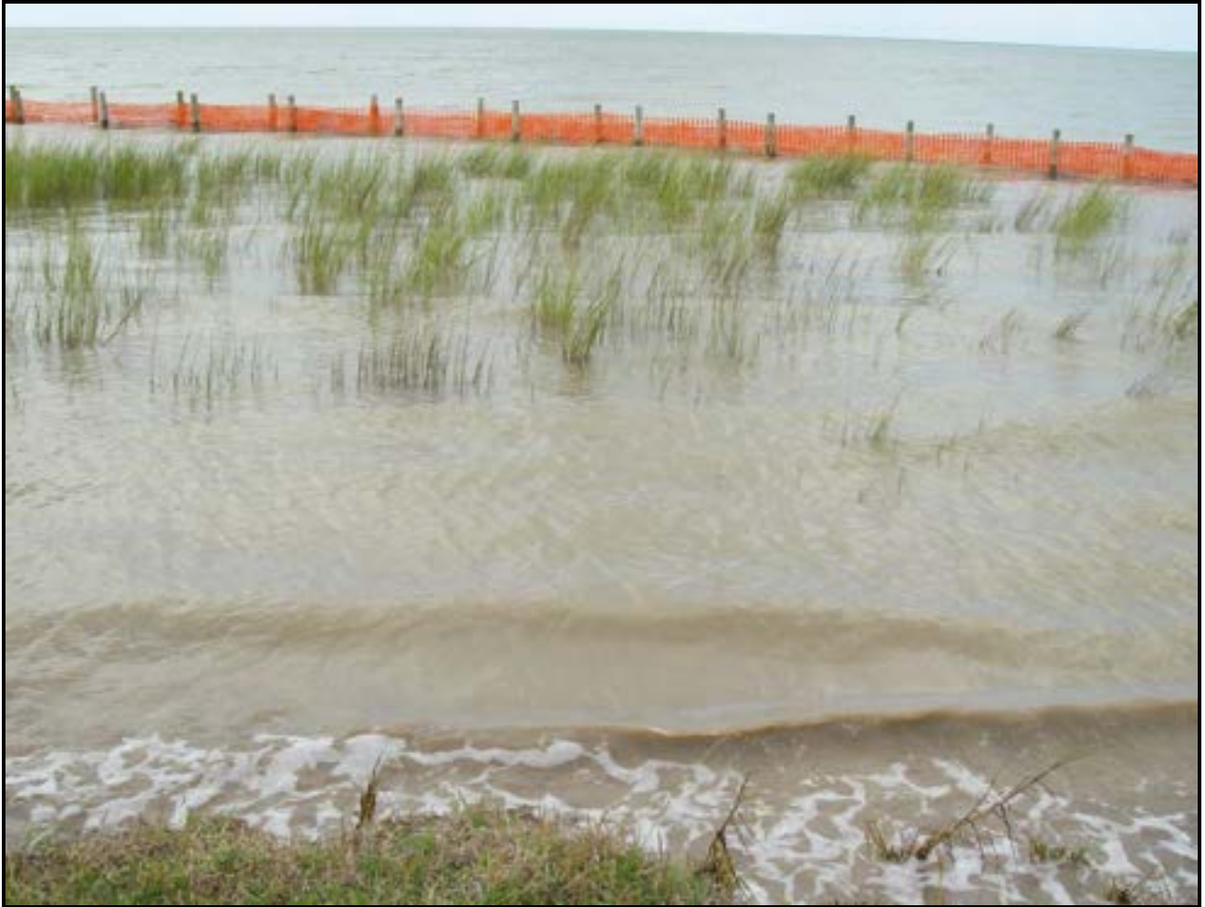
Figure 19. Planting behind erosion control fence
