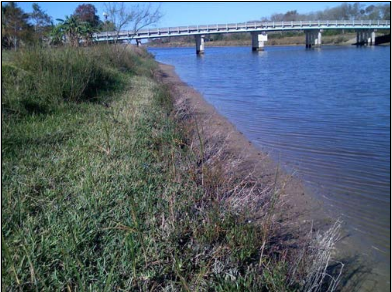
Figure 16. BEFORE: Scarborough shoreline before grading and planting
