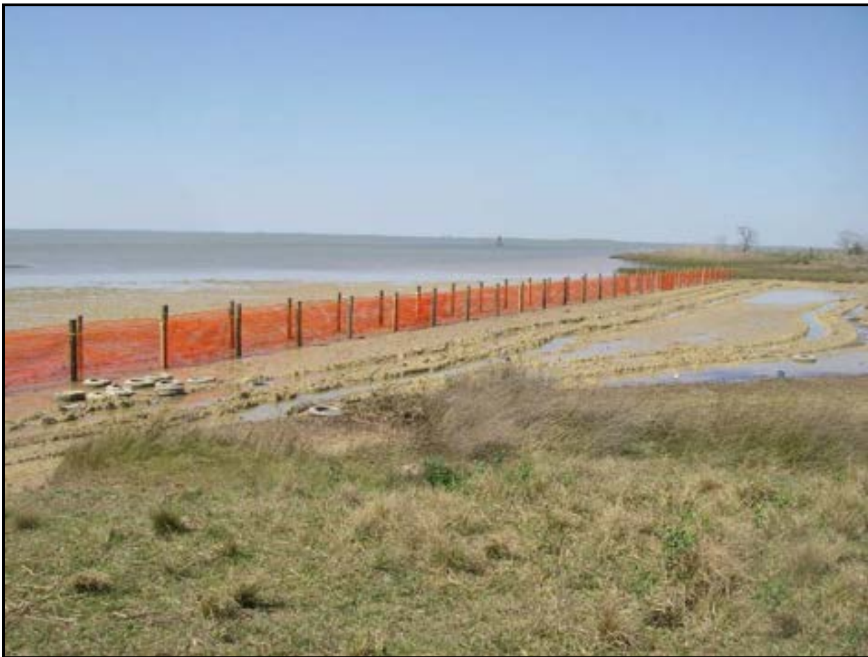
Figure 18. Double-row erosion control fencing
