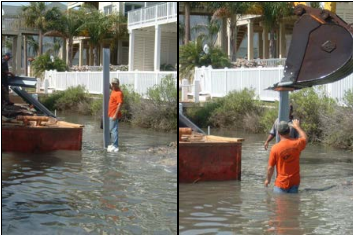
Figure 14. DURING: Vinyl sheetpile installation
