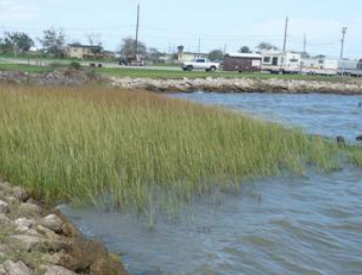
A living shoreline made out of marsh plantings and riprap protect a wooden bulkhead. Photo courtesy of GLO.
