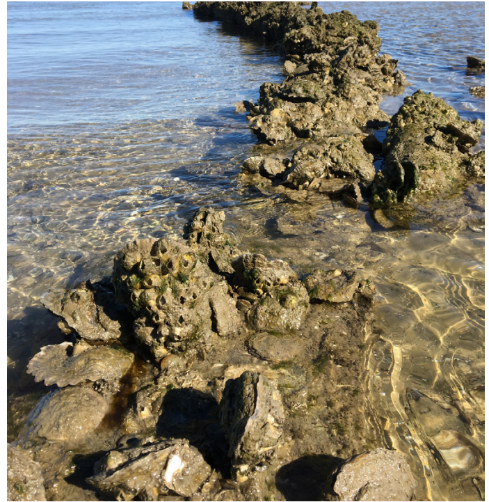
Oyster reef breakwater at Galveston Bay Foundation Sweetwater Preserve property. As oyster conservation efforts ramp up in Texas, there is increased interest in integrating oyster friendly practices into living shoreline design. Photo credit: Galveston Bay Foundation
