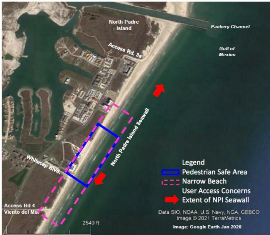
Figure 29. Aerial view of the North Padre Island Seawall and Packery Channel. Erosion at the south end of the Seawall has created difficulties in managing public access.
