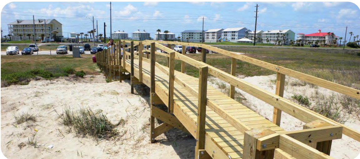
Figure 10. Dune walkover completed following Hurricane Ike.
