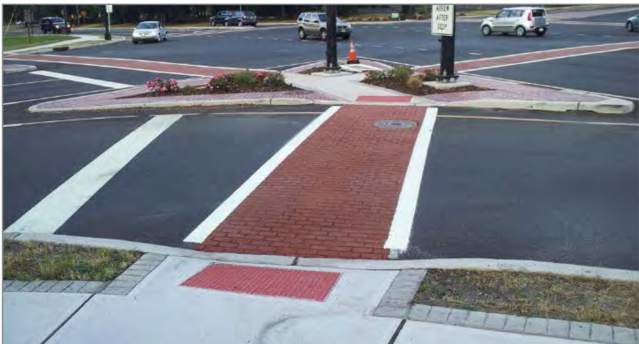
Figure 6-12: Pedestrian crossing constructed with pervious pavers.
