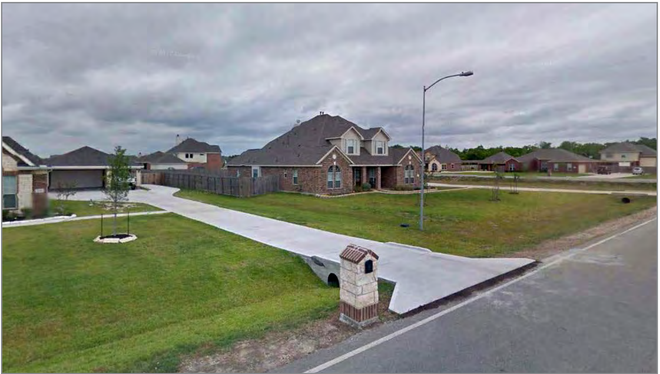
Figure 5-1: Typical swale in a residential neighborhood in Chambers County, Texas. (Photo courtesy of Google Earth)
