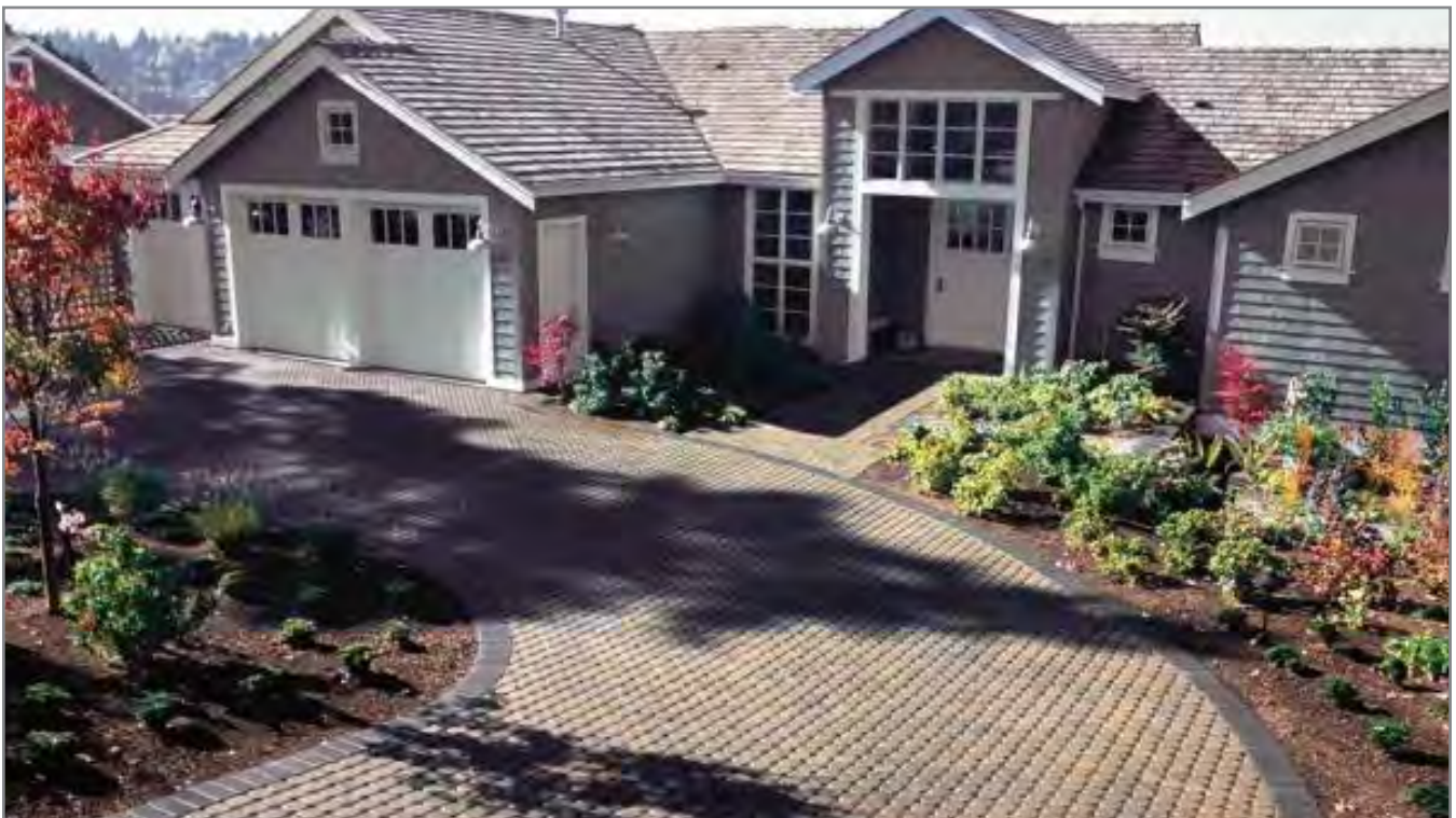
Figure 4-4: Driveway constructed of permeable pavers. (Photo courtesy of Mutual Materials)
