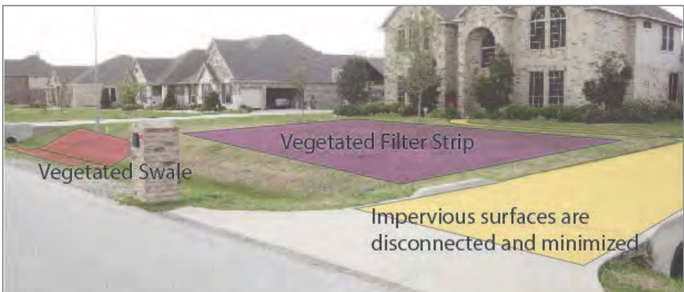
Figure 4-2: Medium density neighborhood uses vegetated swales for stormwater conveyance. These swales also provide water quality benefits.
