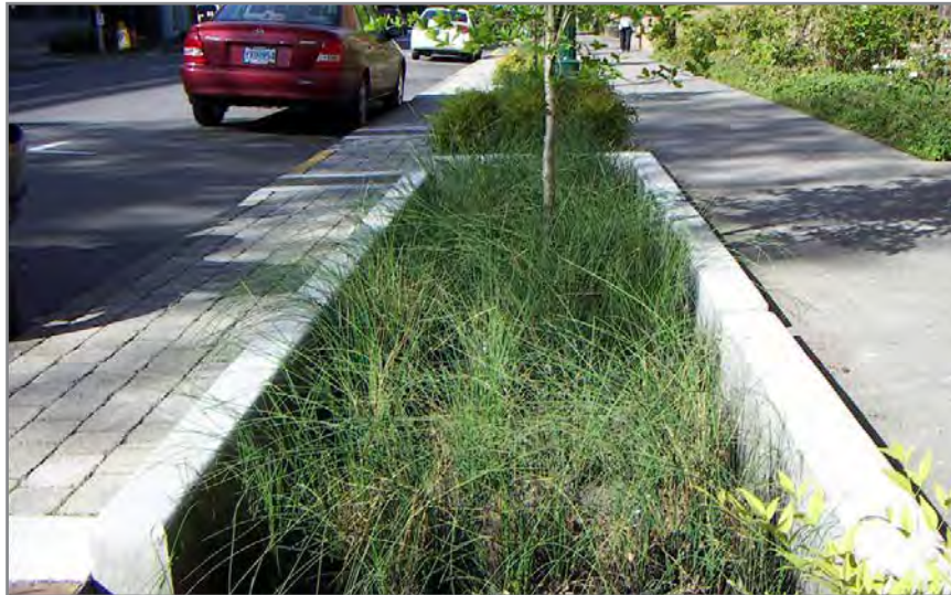
Figure 6-9: Bioretention serves as a buffer between the sidewalk and street. (Photo courtesy of State of Washington Transportation Improvement Board)
