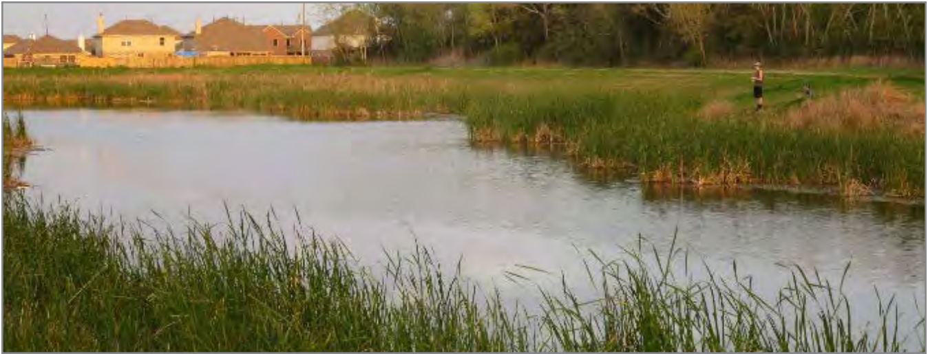
Figure 6-6: Enhanced detention wet pond is an amenity (in a subdivision in Chambers County, Texas).
