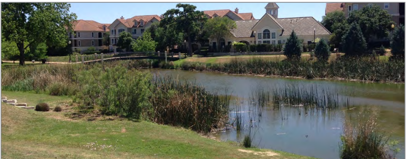
Figure 6-8: Constructed wet pond provides water quality benefits and an attractive place to recreate for nearby multi-family housing.
