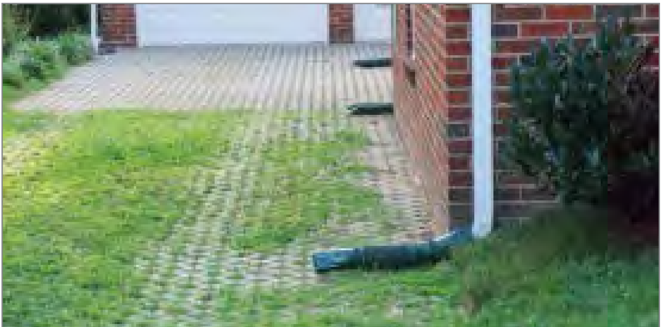
Figure 2-5: Downspouts directed to permeable pavement on driveway. (Photo courtesy of Montgomery County, Maryland)
