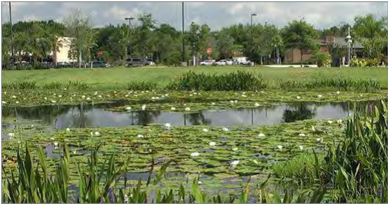
Figure 5-8: Picture of an enhanced detention wet pond. (Photo courtesy of Houston-Galveston Area Council)
