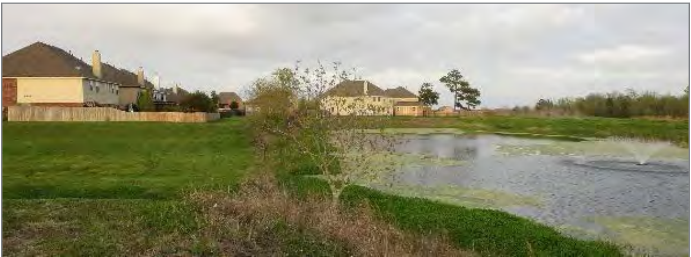
Figure 6-7: Chambers County neighborhood uses wet pond with a fountain for water circulation as a prominent feature in the subdivision.
