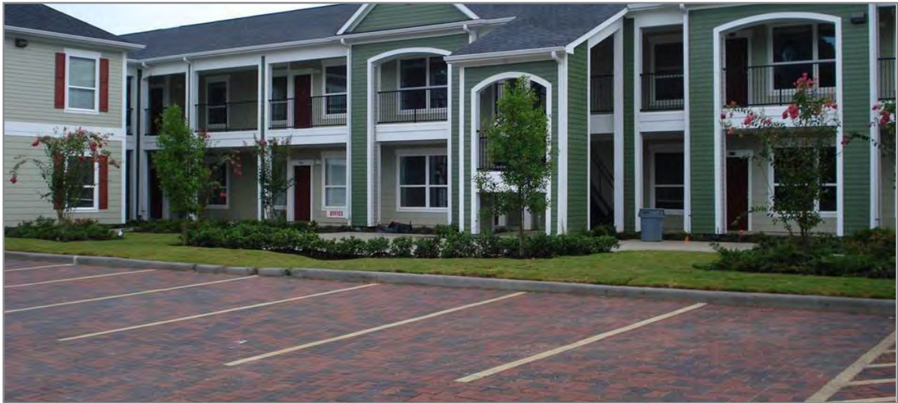
Figure 4-7: Multi-family units utilize permeable pavers to beautify their parking lot
