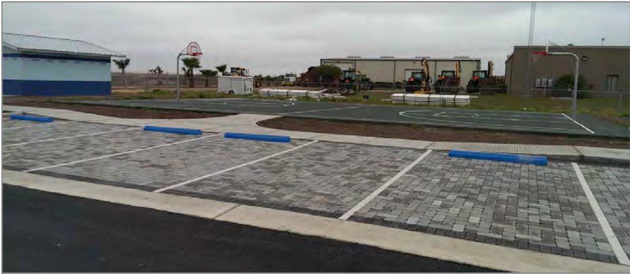
Figure 5-5: Permeable pavers in parking stall of Cascade Park parking lot in Cameron County.
