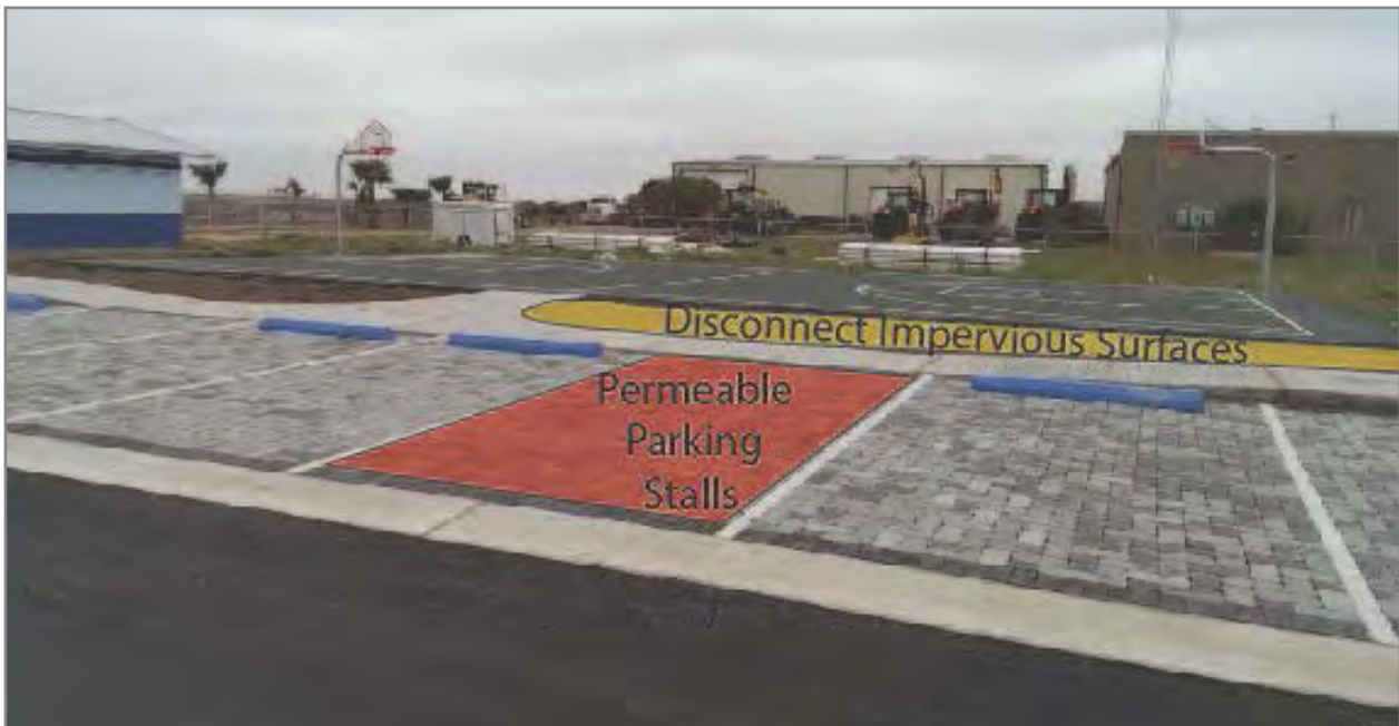
Figure 4-10: Permeable interlocking concrete pavers with regular asphalt driving lane in Cascade Park parking lot, Cameron County, Texas.
