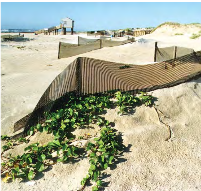
Figure 17. Sand fencing used to trap sand.
