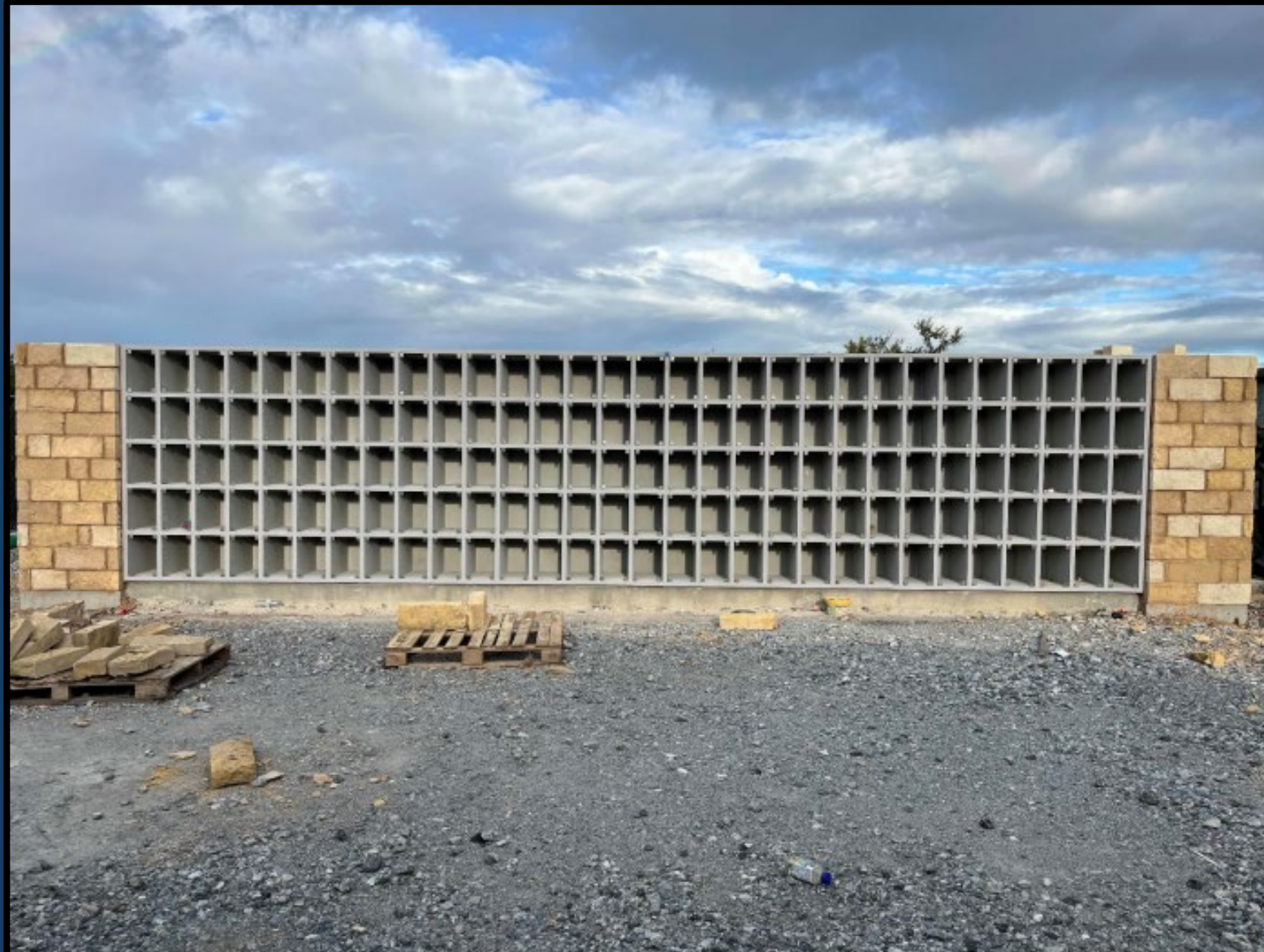
Columbaria Plaza – Double Sided wall masonry veneer installation.
