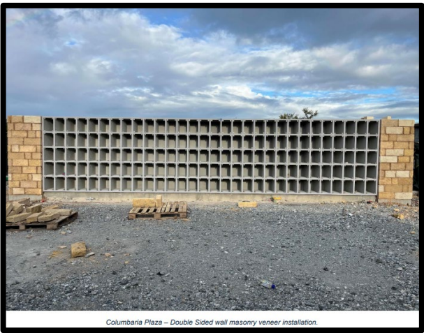
Columbaria Plaza – Double Sided wall masonry veneer installation.
