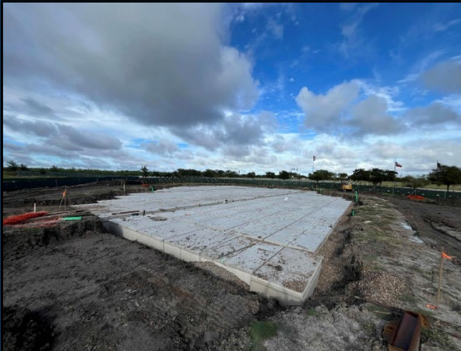
Section 7 – Completed crypt placement.
