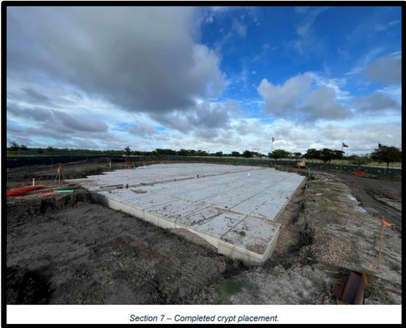
Section 7 – Completed crypt placement.
