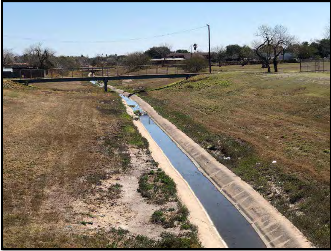
Tranquitas Creek Existing Channel
