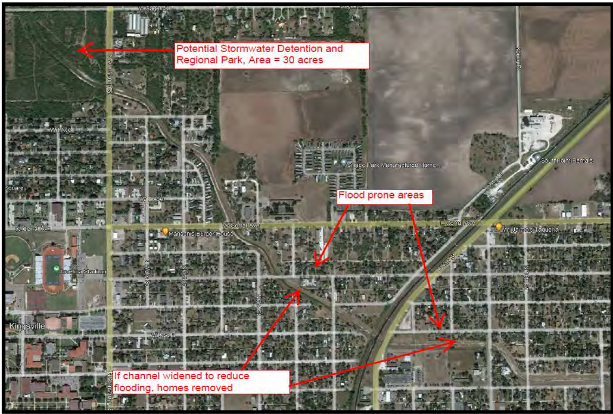
Tranquitas Creek Regional Detention Site (upper left)
