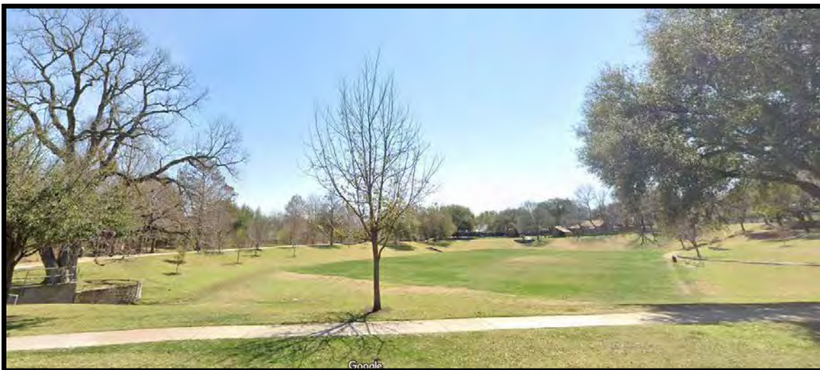
Extended Detention Basin with Soccer Field
