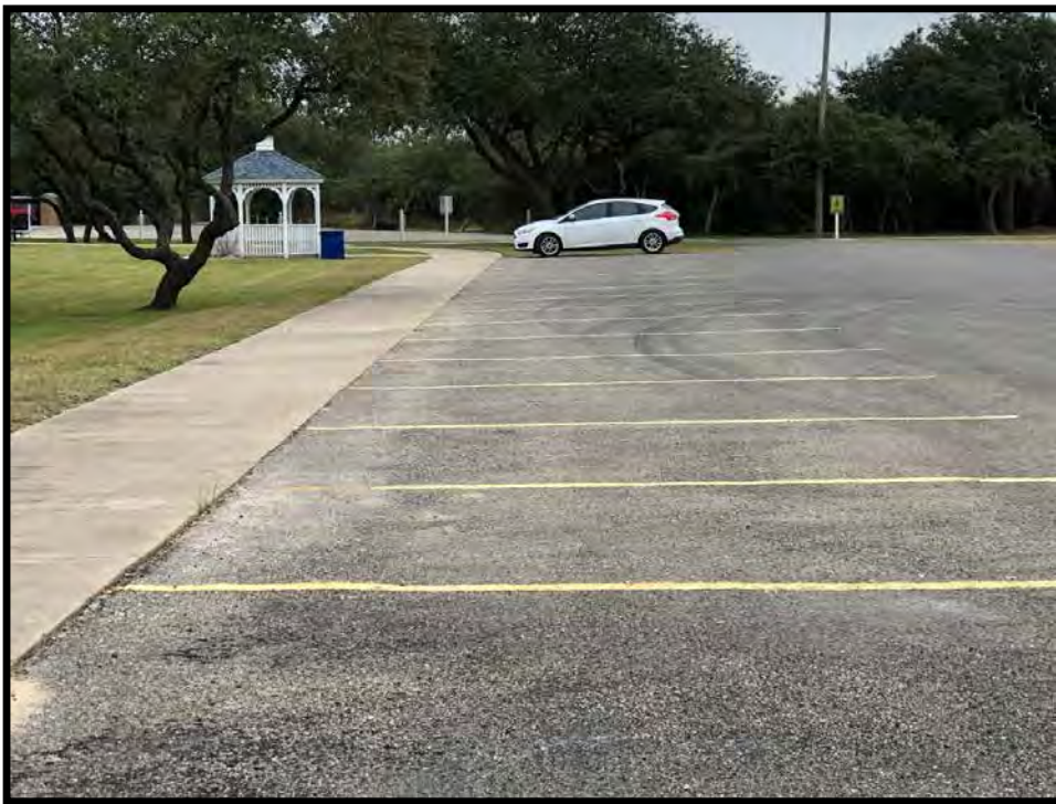
Rockport Aquatic Complex Parking Lot
