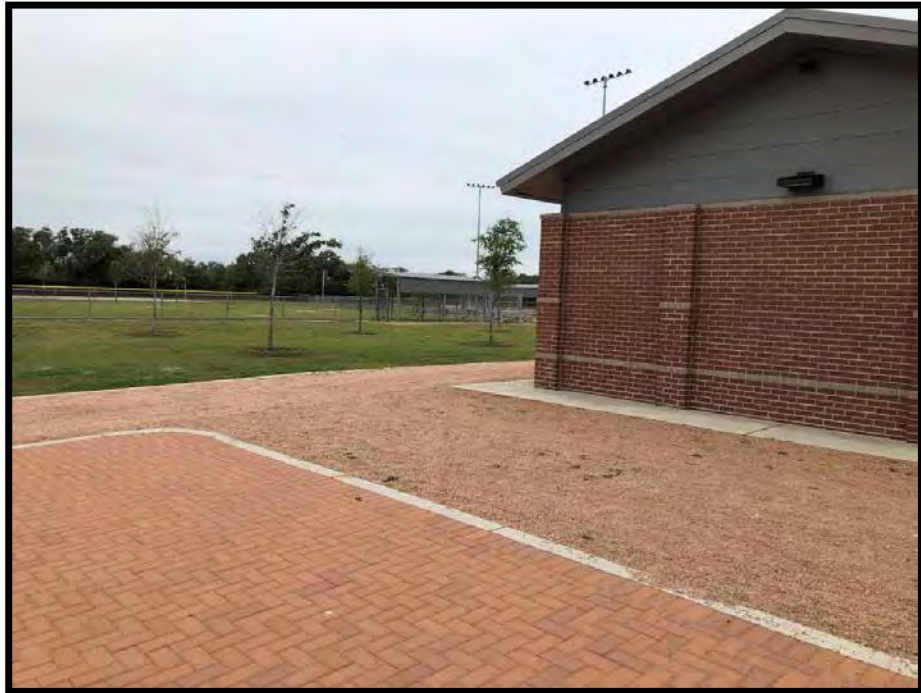
Rockport Memorial Park Building to be Retrofit with a Rainwater Harvesting Tank
