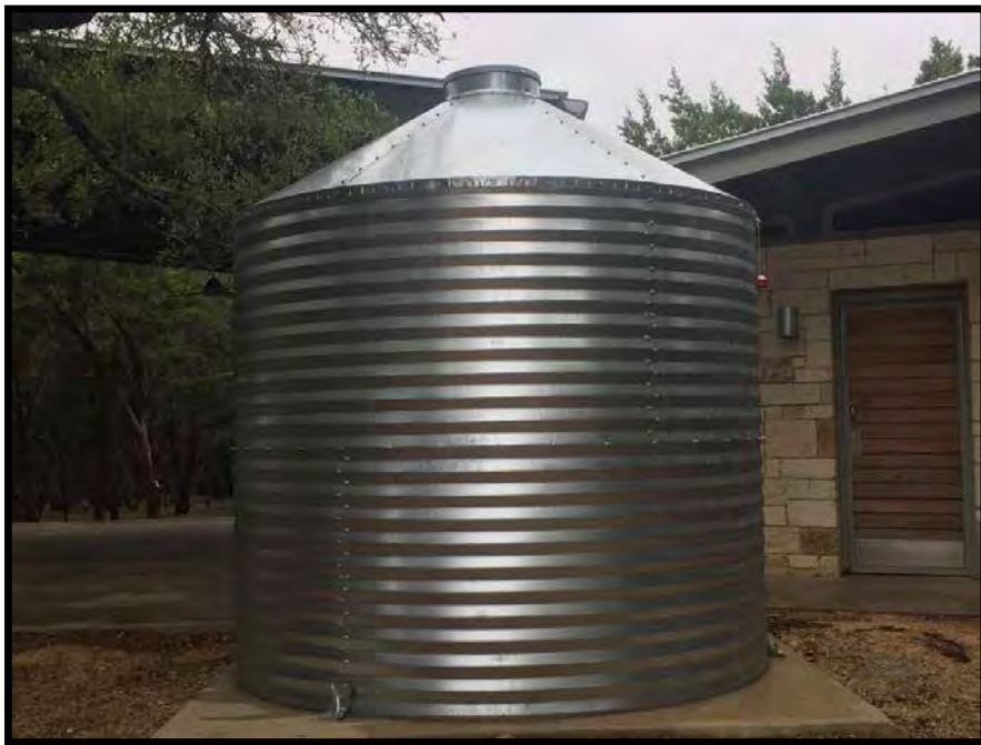
Rainwater Harvesting Tank
