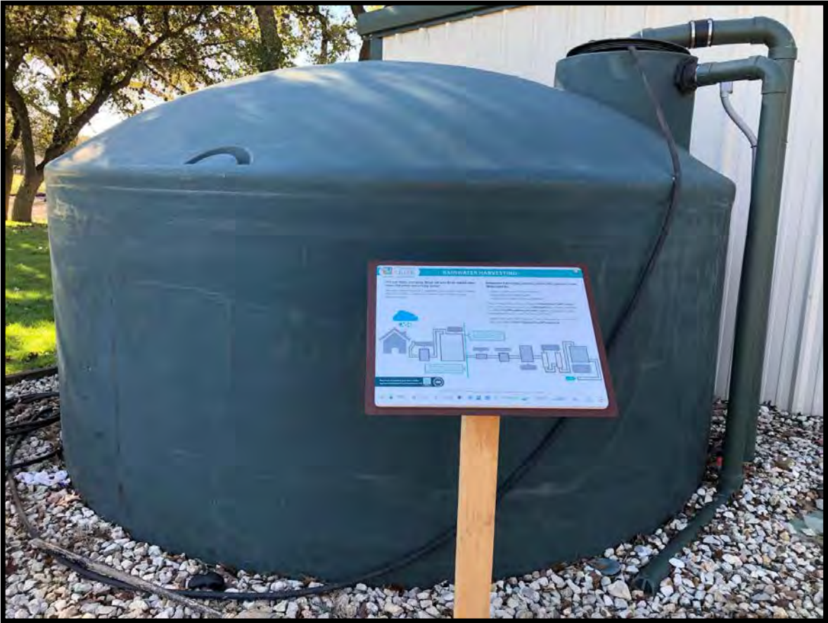
Figure 2-Woodcreek Golf Course Rainwater Harvesting
