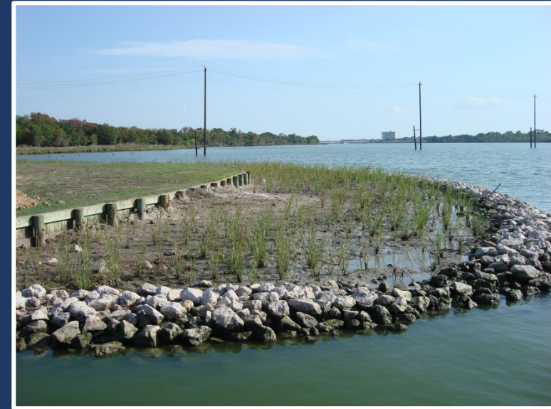
Retrofit: Hybrid Stabilization
