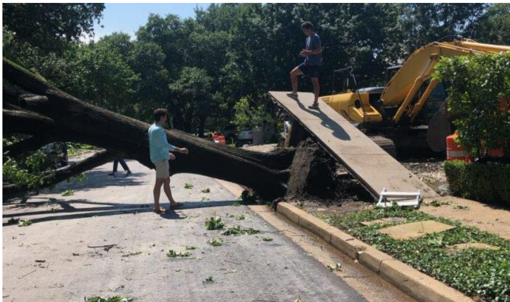
Figure 3-52: Uprooted tree-damaged sidewalk infrastructure and blocked roadway in Dallas, June 2019, following severe winds associated with thunderstorms. 253
