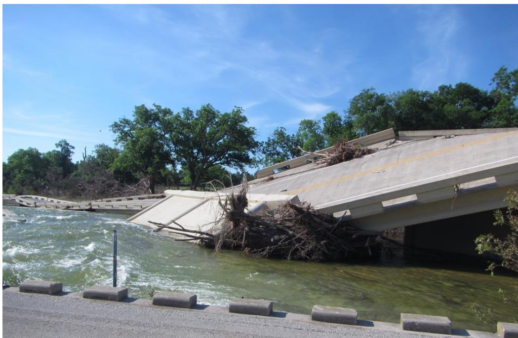
Figure 3-1: Fischer Store Road Bridge Over the Blanco River 4
