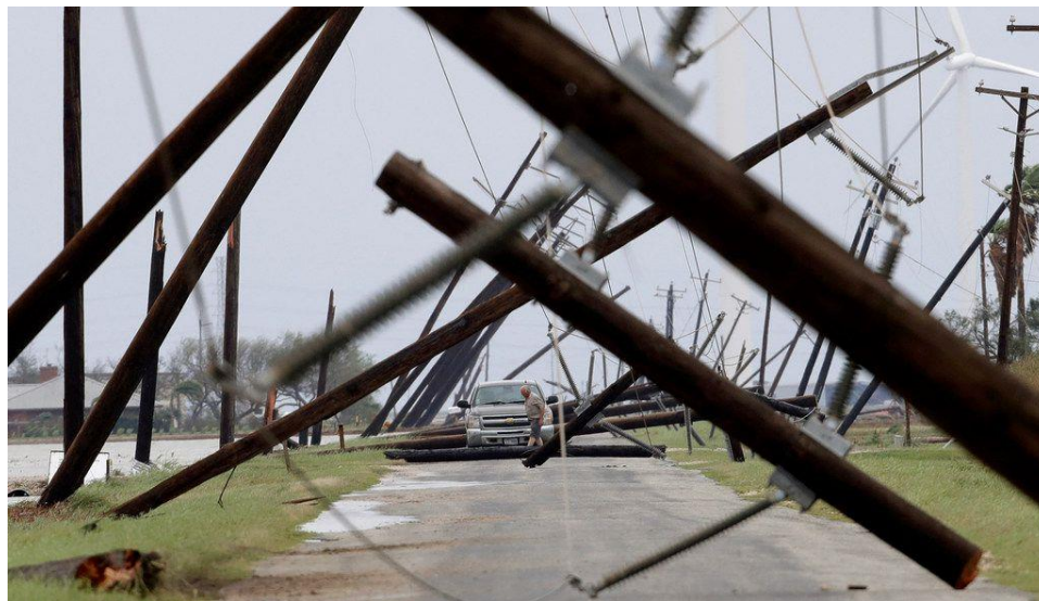
Figure 3-32: Downed utility lines near Taft, Texas, during Hurricane Harvey. 125
