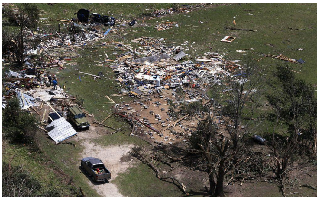
Figure 3-49: Destroyed home in Canton, April 2017 tornadoes. 237
