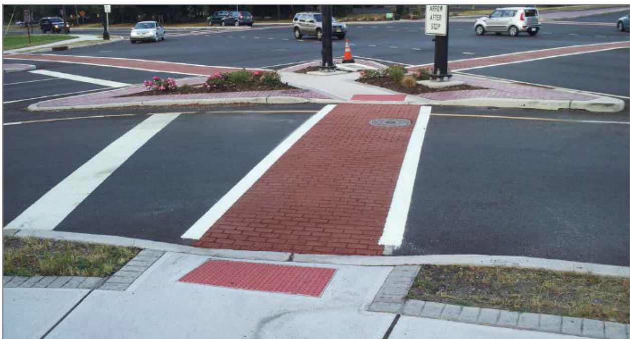
Figure 6-12: Pedestrian crossing constructed with pervious pavers.
