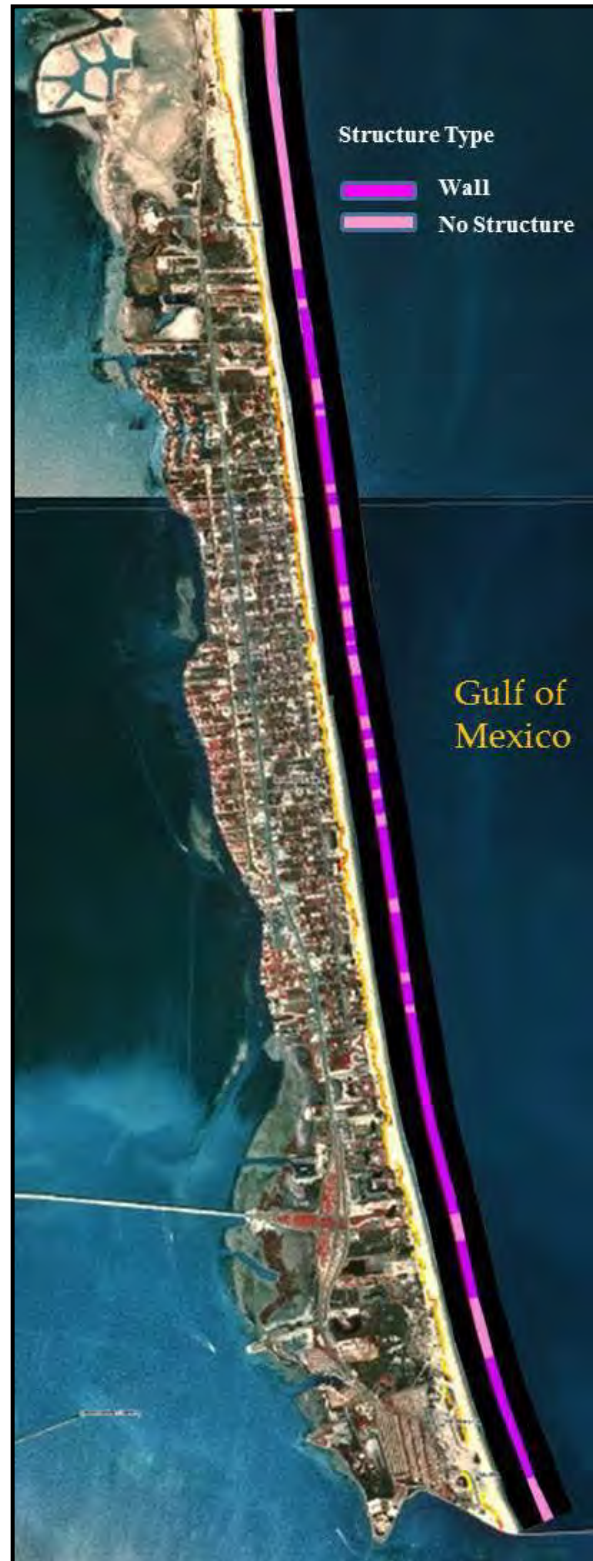
Figure 25 Modified coastal classification scheme from Morton and Peterson (2006). Much of the shoreline along the developed portion of SPI has retaining walls
