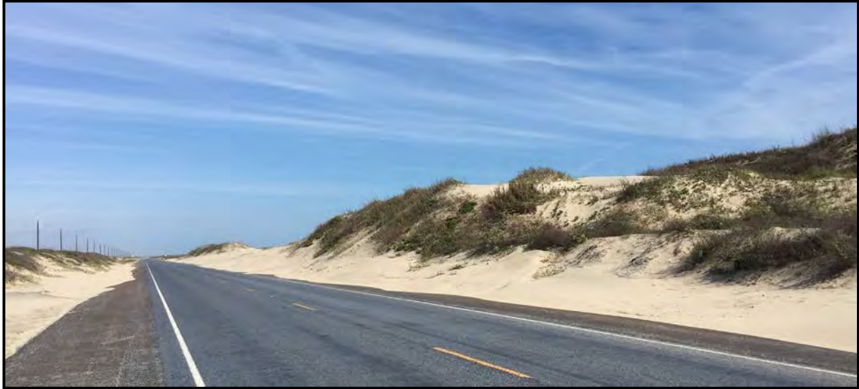
Photo 2: Park Road 100. Note sand adjacent to the road. By Jeb Boyt
