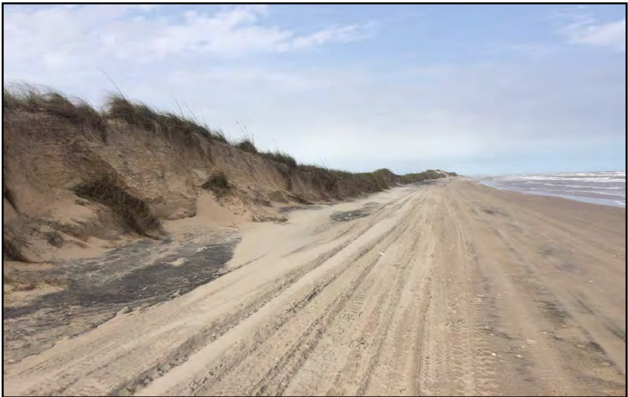
Photo 1: Example of eroding dune scarp in Zone 3. By Peter Ravella, March 2016
