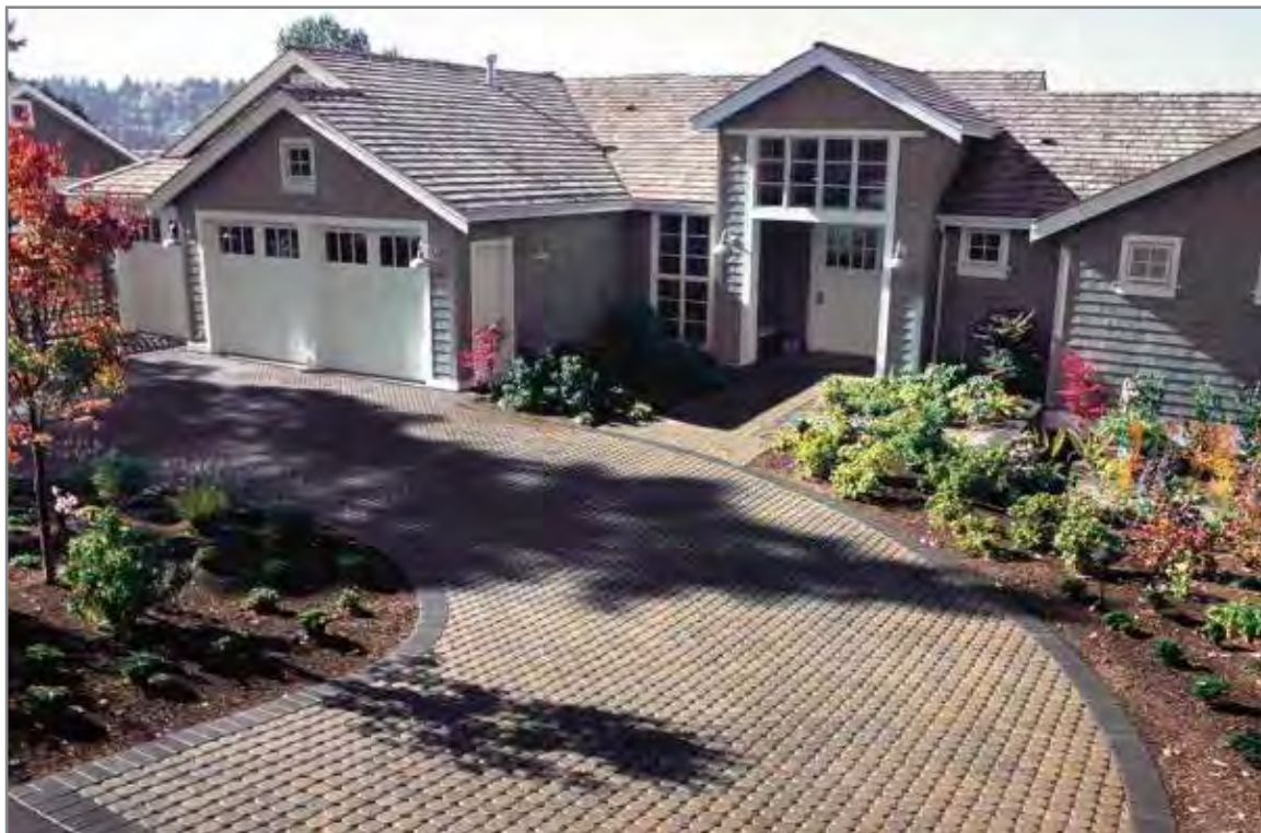
Figure 4-4: Driveway constructed of permeable pavers. (Photo courtesy of Mutual Materials)
