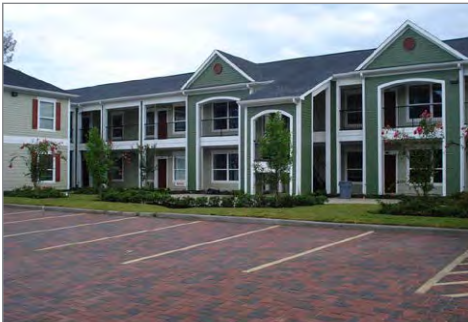
Figure 4-7: Multi-family units utilize permeable pavers to beautify their parking lot.
