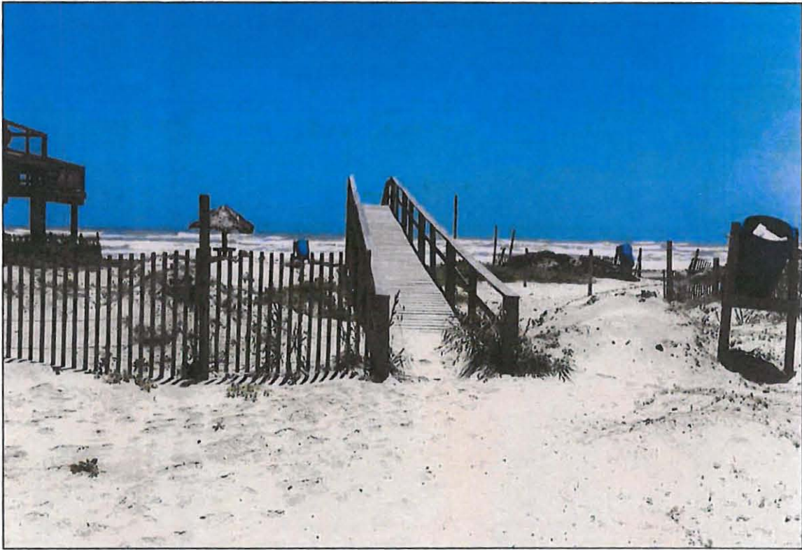
(K.) Village of Surfside Beach: Pedestrian Beach Access Point at Francis Cove. (IMG_0664.JPG)
