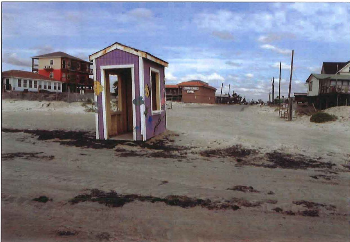
(L.) Village of Surfside Beach: Vehicle Beach Access Point at Ocean Ave. (DSCF0138.JPG)
