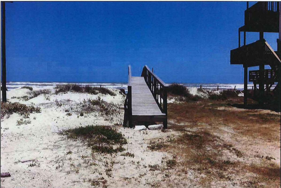
R. Village of Surfside Beach: Pedestrian Beach Access Point at Howard Ave. (IMG_0680.JPG)
