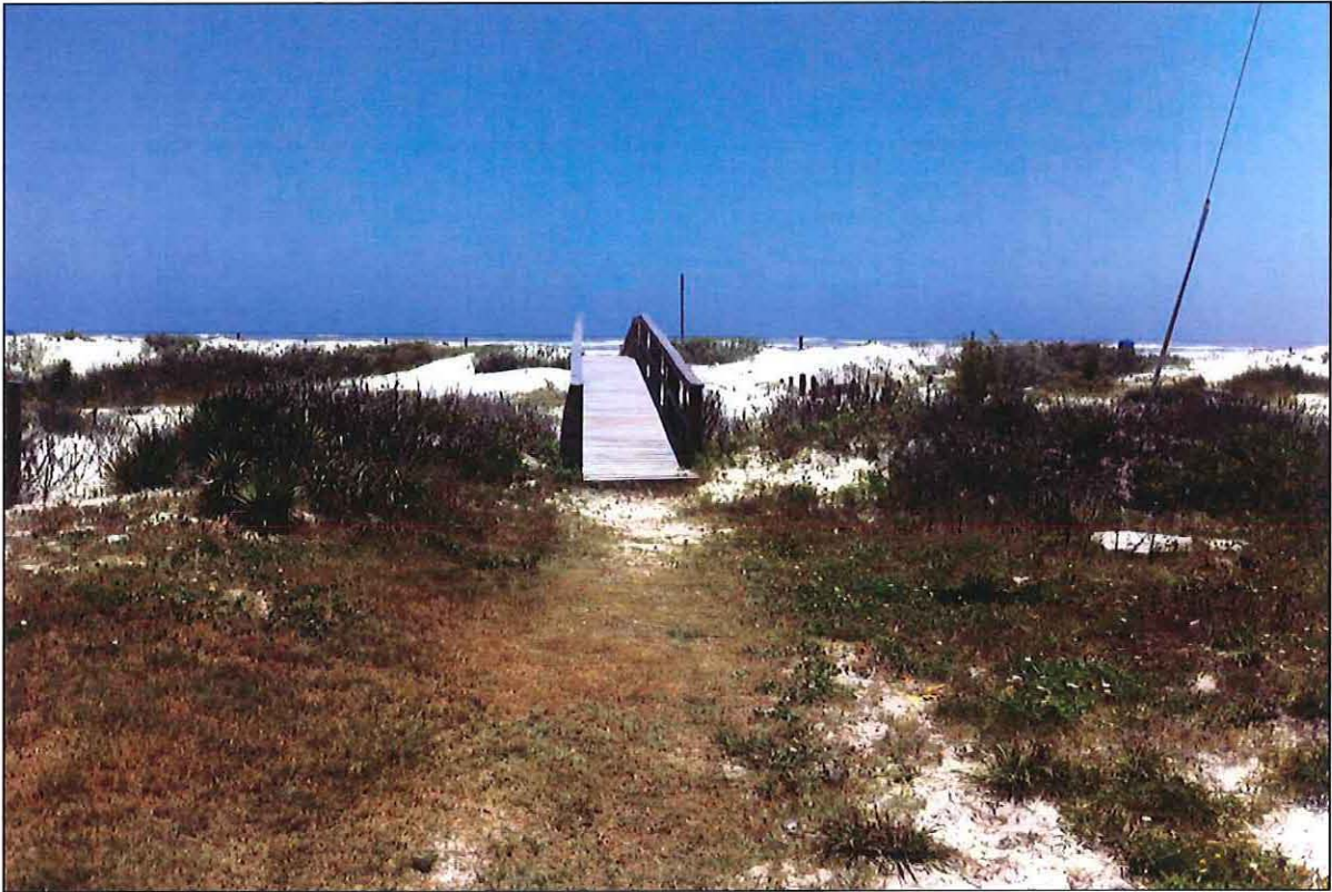
U. Village of Surfside Beach: Pedestrian Beach Access Point at Detenbeck Ave. (IMG_0686.JPG)
