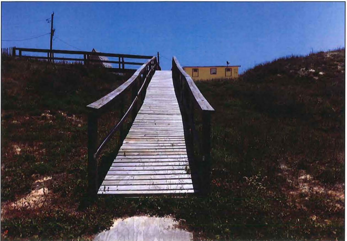
(P.) Village of Surfside Beach: Pedestrian Beach Access Point at Gulfway Ct. (IMG_0674.JPG)
