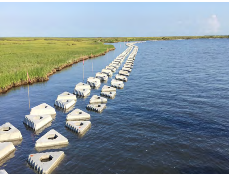
Breakwater of Precast Concrete Forms. Photo: Mott MacDonald
