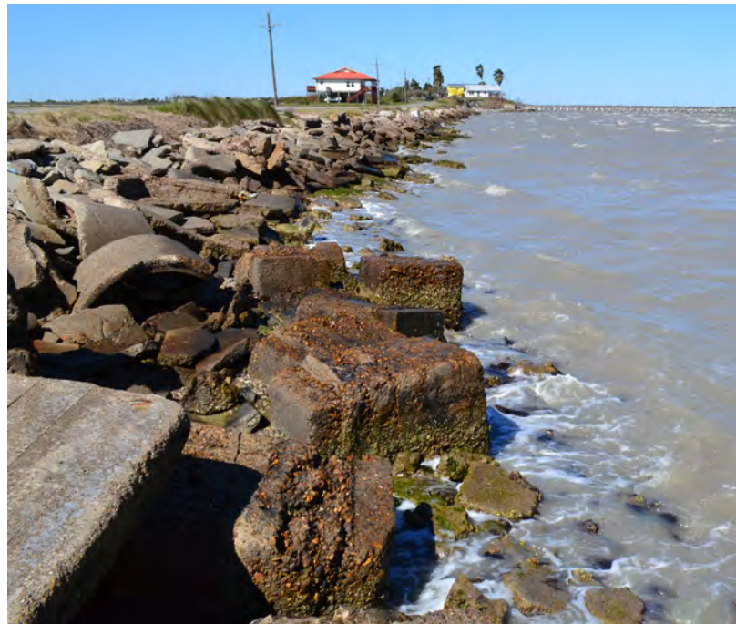
Riprap Only Shoreline. Photo: Texas General Land Office
