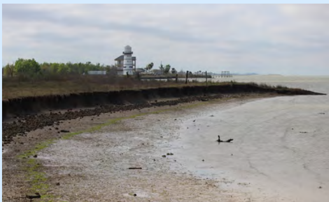
Shoreline Erosion. Photo: Galveston Bay Foundation
