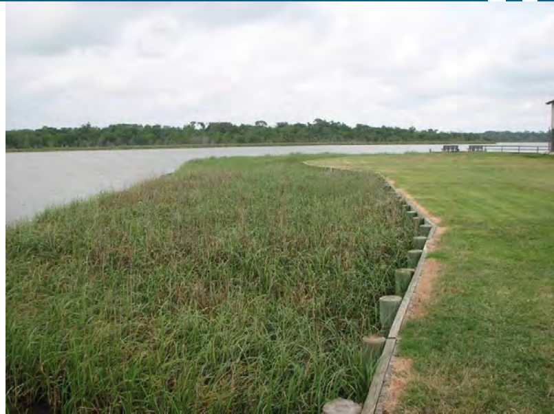
Limestone Breakwater with Marsh Planting Installation - After. Photo: Galveston Bay Foundation
