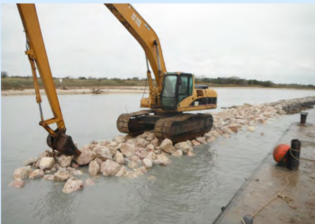
Riprap Installation. Photo: Mott MacDonald
