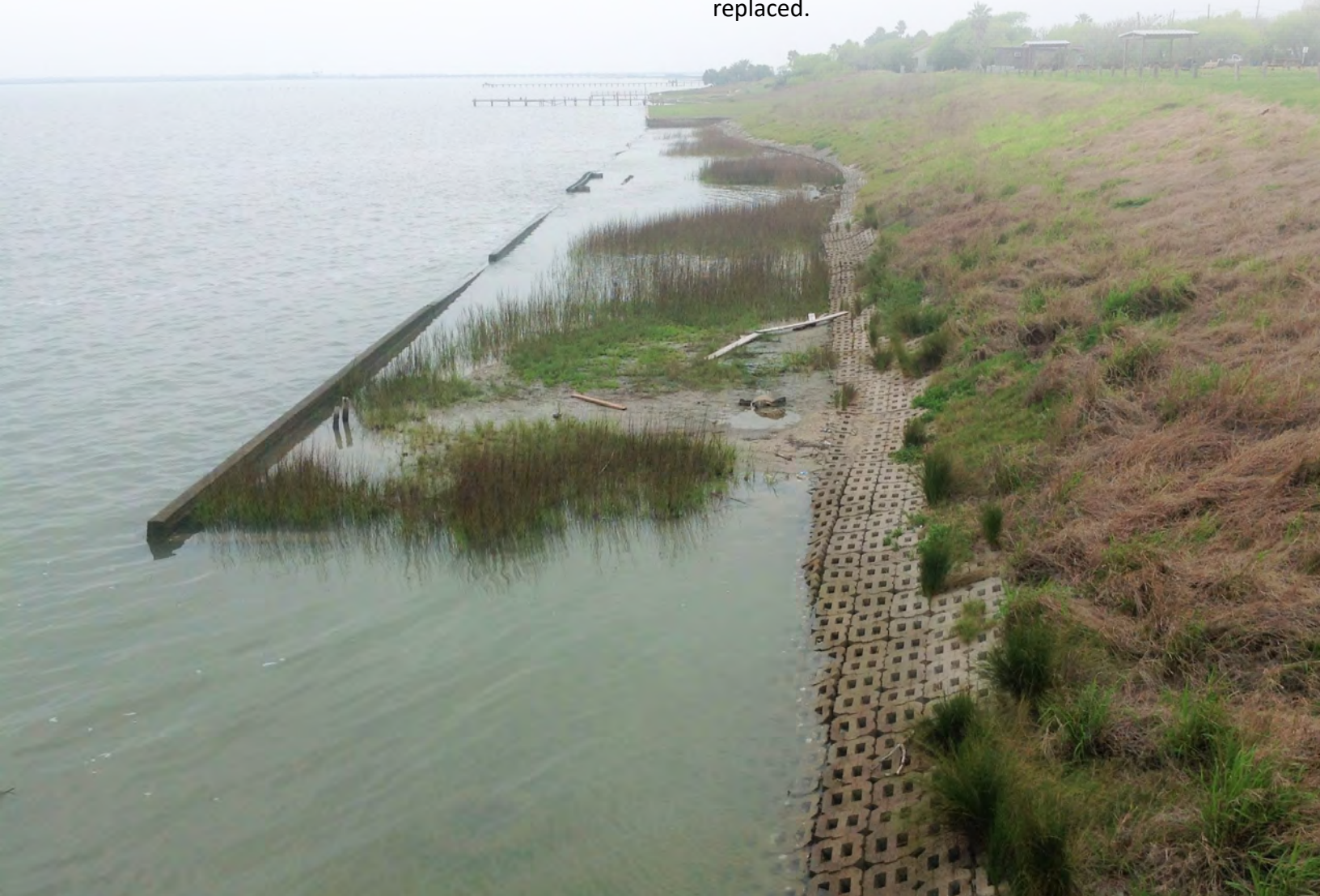
Articulated Mats Stabilizing Vegetation as Part of a Living Shoreline Project. Photo: Texas General Land Office
