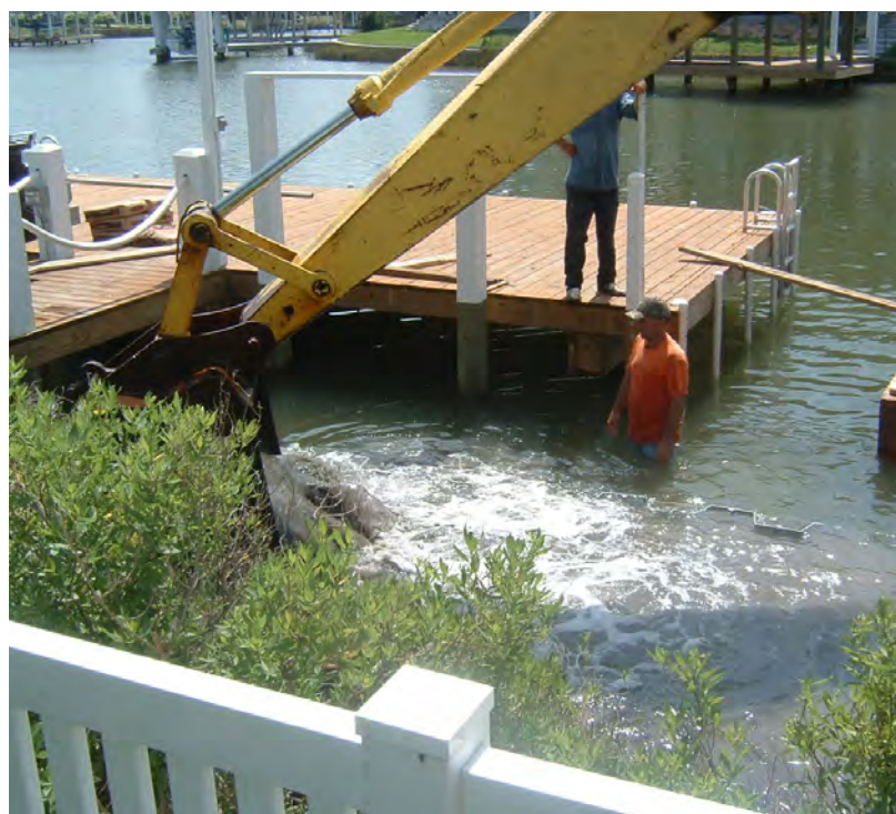
Construction of a Restored Marsh Habitat. Photo: Galveston Bay Foundation
