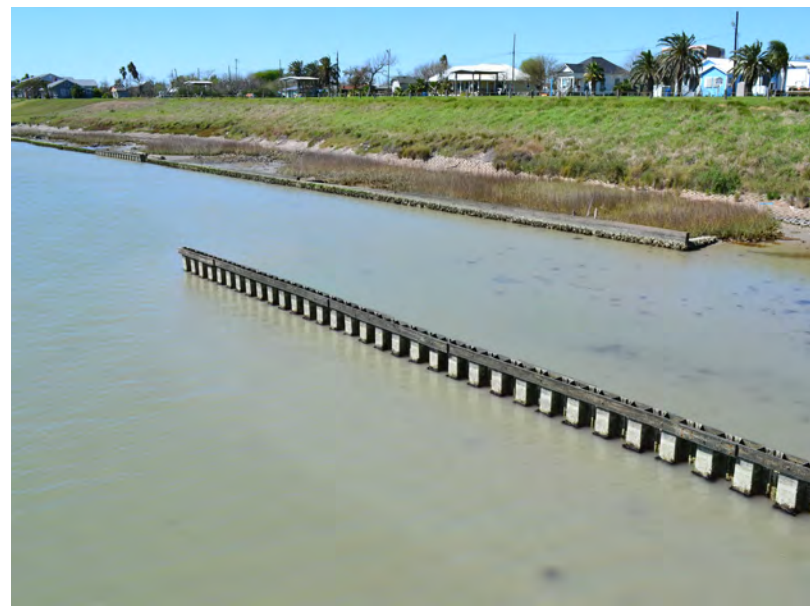
Vinyl Sheet Pile Breakwater. Photo: Texas General Land Office
