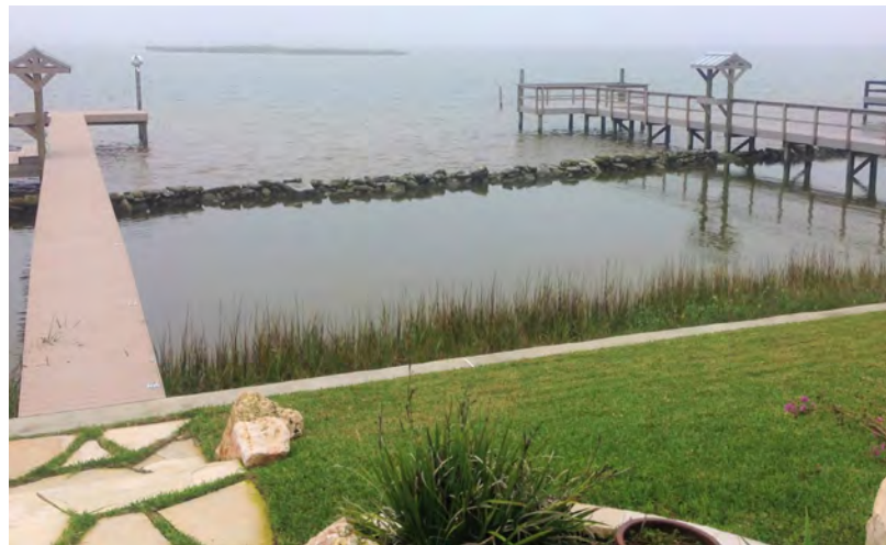
Rock Rubble Breakwaters Protecting Area of Planted Seagrass (Under the Water) and Cordgrass Along the Bulkhead. Photo: Texas General Land Office
