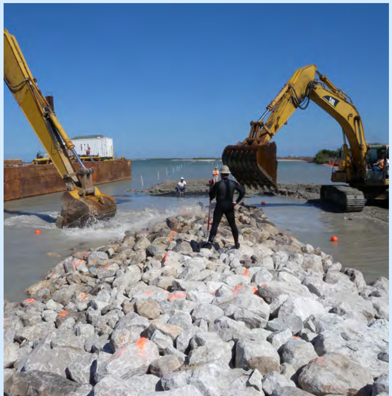
Riprap Installation. Photo: Mott MacDonald
