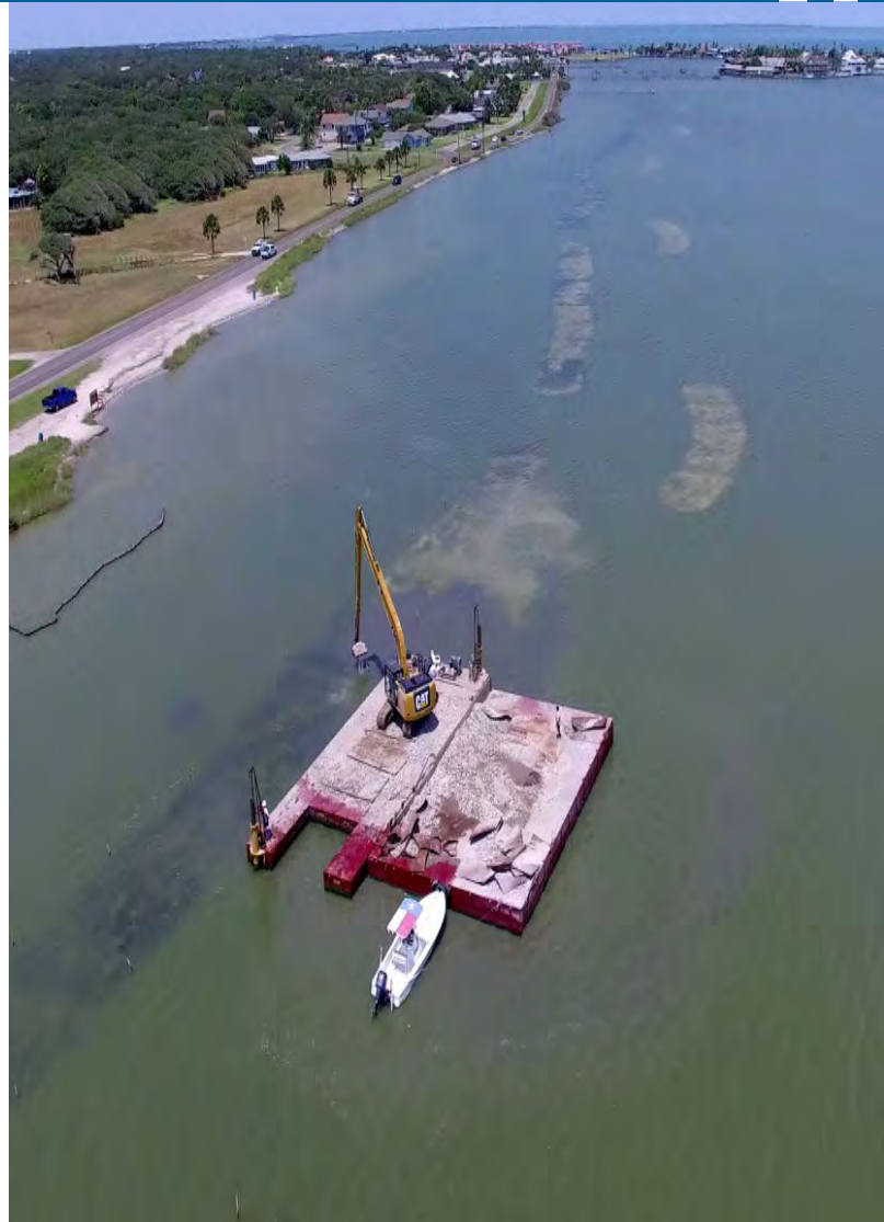
Submerged Oyster Shell Bed Installation Little Bay, Rockport, Texas. Photo: AECOM
