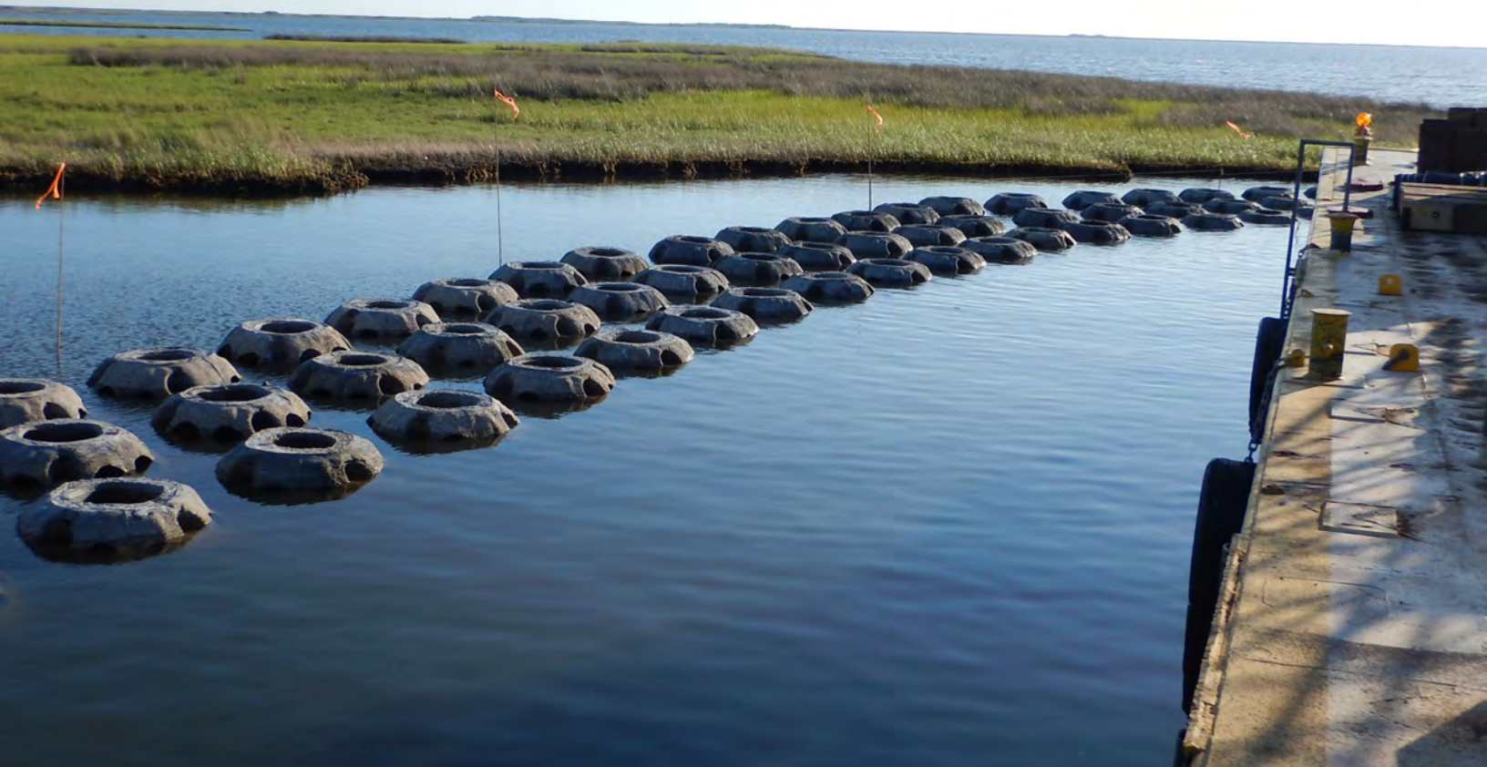
Reef Ball Installation. Photo: Mott MacDonald
