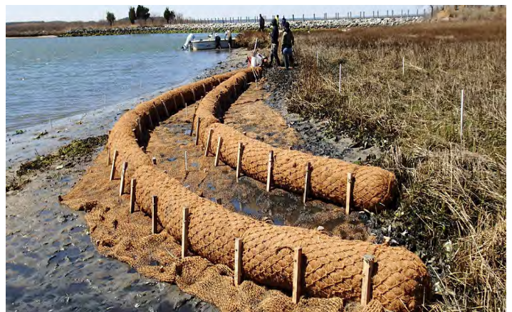
Coir Log Installation. Photo: Delaware Living Shorelines
