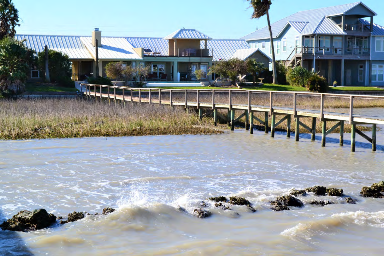
Living Shoreline with Marsh Planting and Breakwater. Photo: Texas General Land Office
