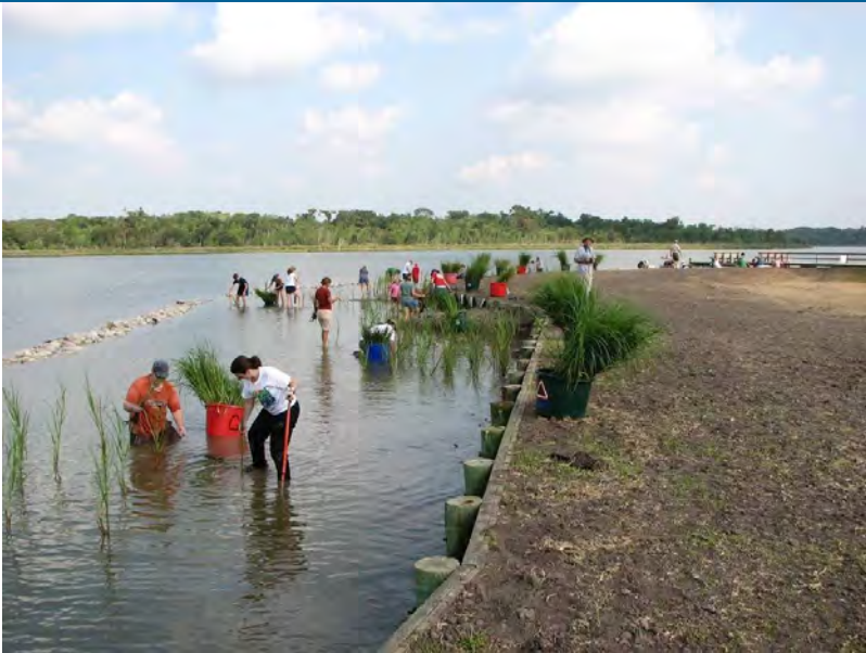
Limestone Breakwater with Marsh Planting Installation - Before. Photo: Galveston Bay Foundation
