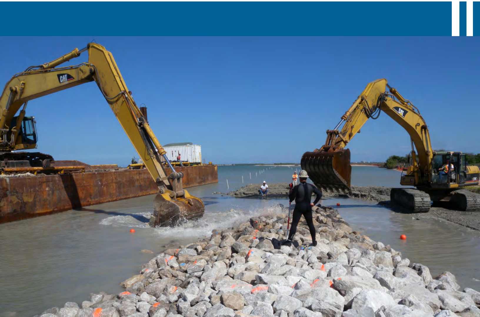
Riprap Breakwater Installation. Photo: Mott MacDonald
