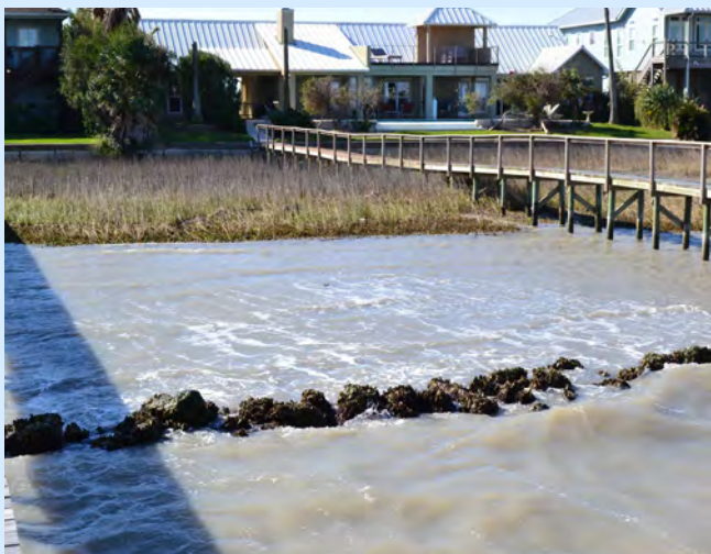
Rock Rubble Breakwater with Oysters Attached. Photo: Texas General Land Office
