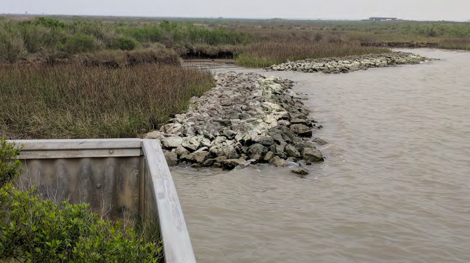
Segmented Breakwater with Marsh Plantings. Photo: AECOM
