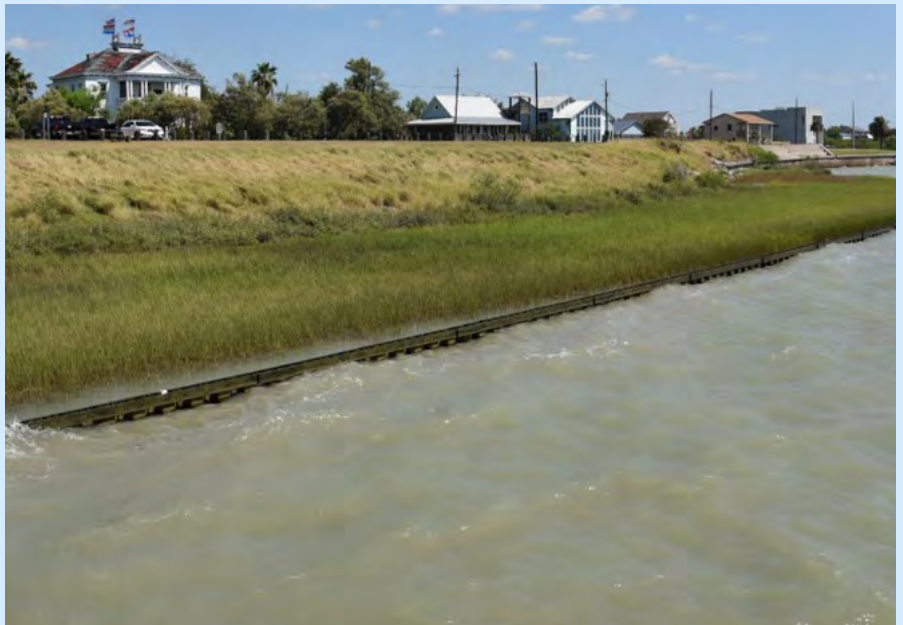
Photo: Coastal Bend Bays and Estuaries Program
