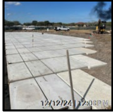
Section 10 crypt installation
