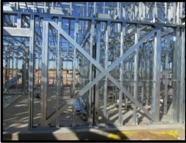
Admin building steel frame
