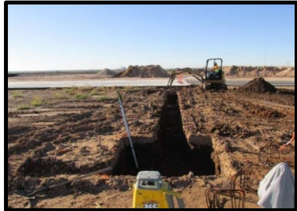
Footings for Maintenance building
