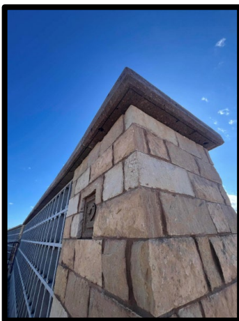
Capstone installation in columbaria
