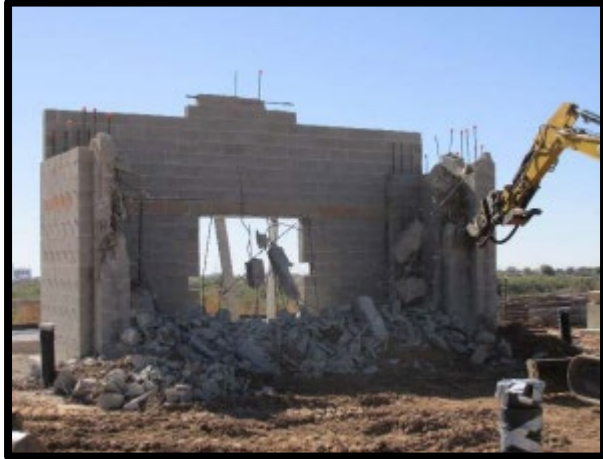
Committal Shelter demolition
