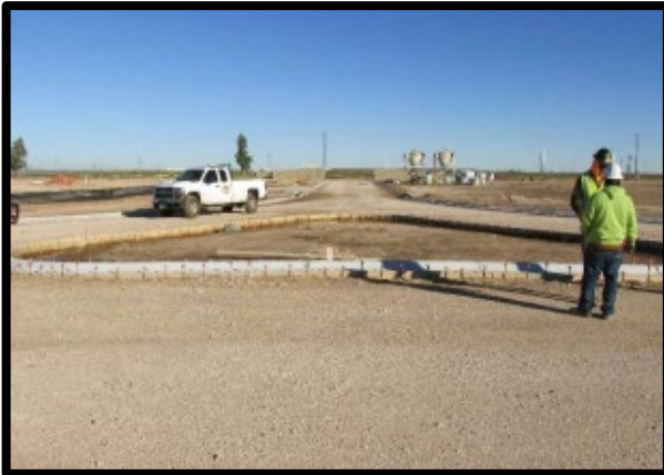
Curbing installed around Texas flag plaza
