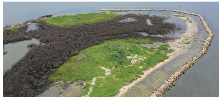
A rock breakwater protects the Dagger Island shoreline and marsh from eroding. The newly planted smooth cordgrass will grow to establish habitat for bird foraging.
