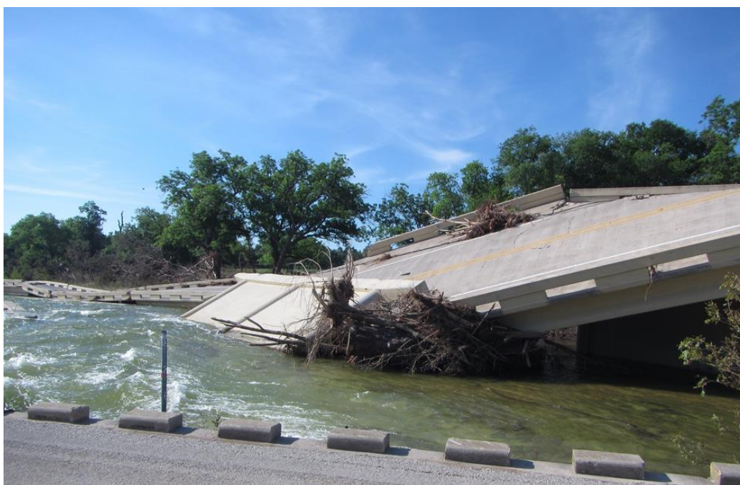
Figure 3-1: Fischer Store Road Bridge Over the Blanco River 4
