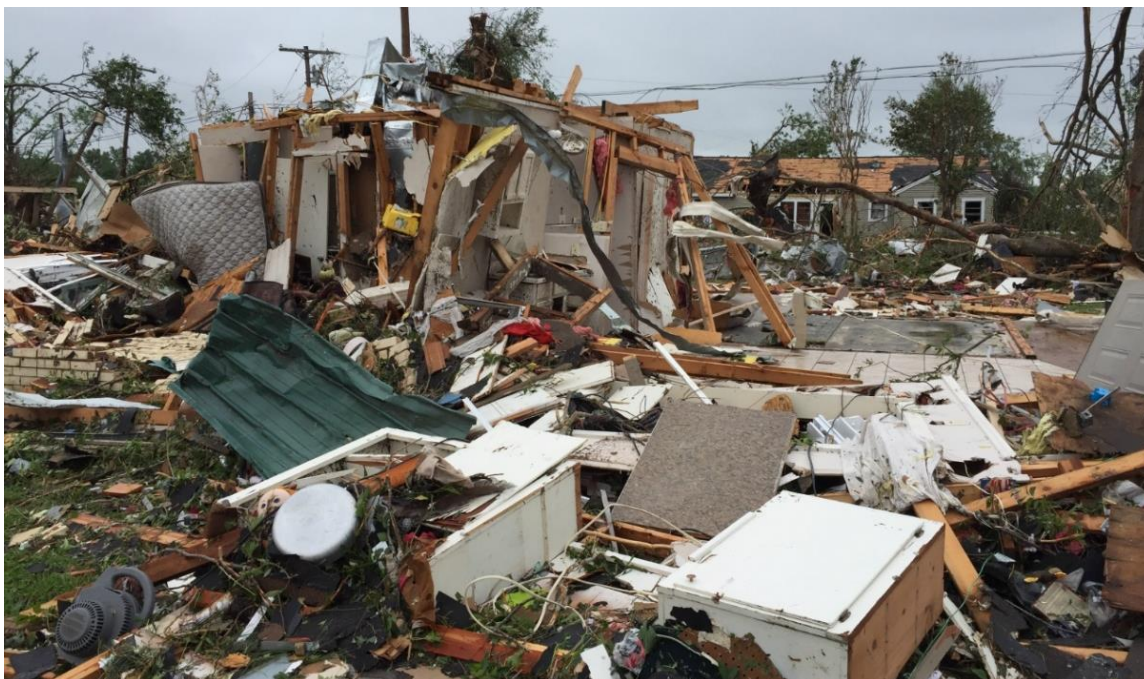
Figure 3-47: Residential neighborhood after EF3 tornado hit Van, Texas, in 2015. 228
