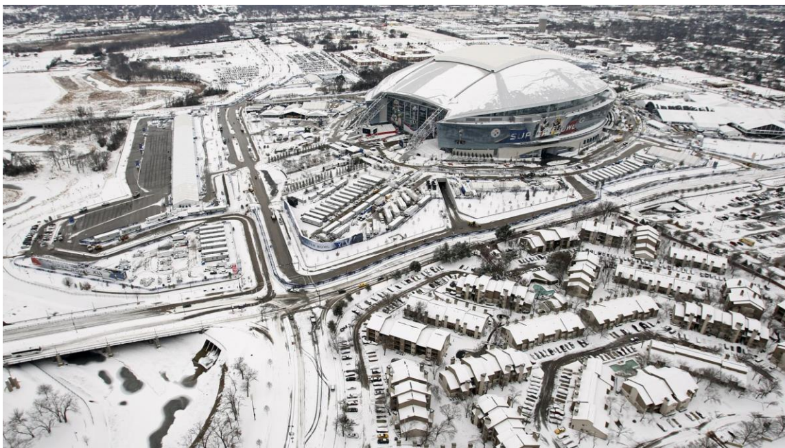
Figure 3-65: Snow and ice covered AT&T Stadium in Arlington, February 2011. 365
