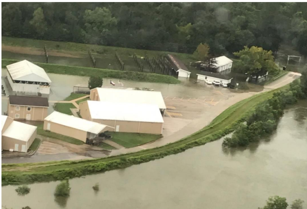
Figure 3-29: City of Conroe’s wastewater treatment plant during Hurricane Harvey. 85
