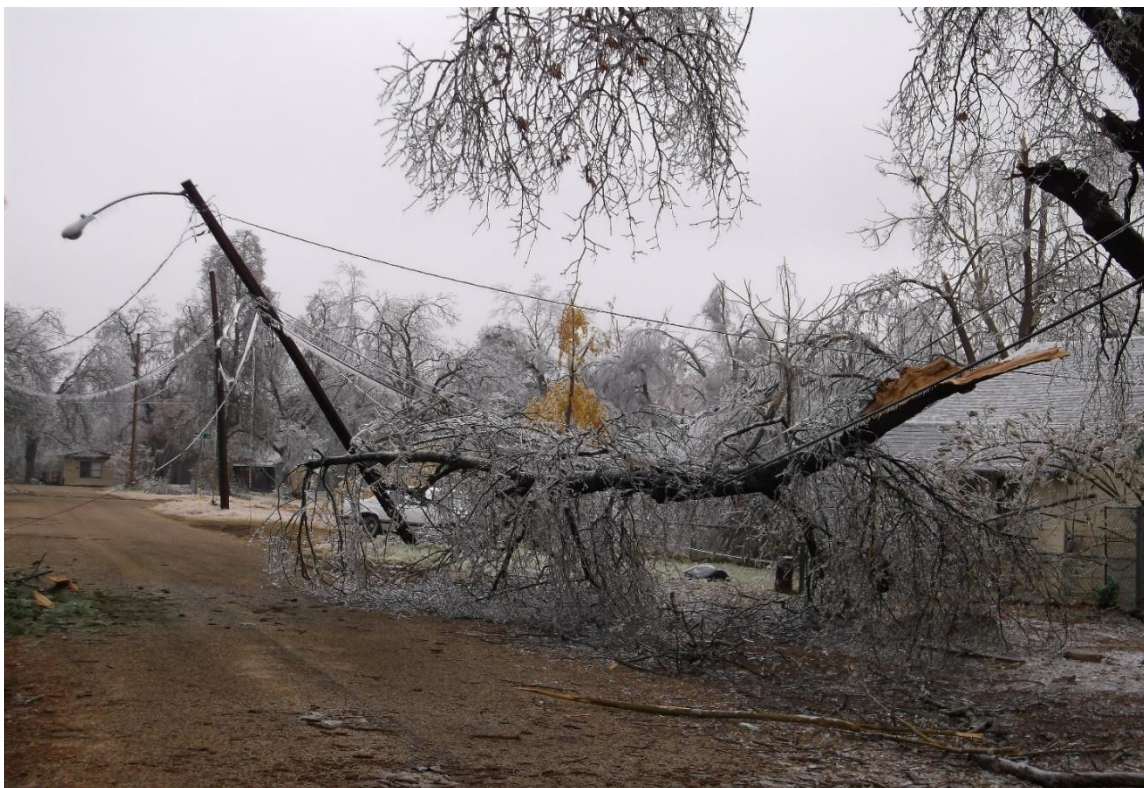
Figure 3-60: Downed power line during the 2013 ice storm in Paris, Texas. 334
