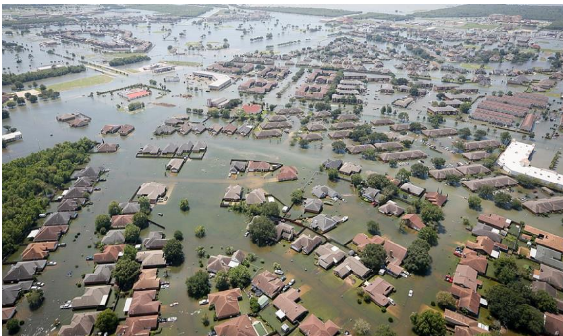
Figure 3-28: Flooding in Port Arthur, Texas, during Hurricane Harvey. 75
