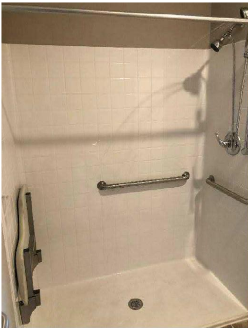
HC-4 Roll-In Shower with Grab Bars, Fold-up Seat, and Shower Wand (ADA Compliant)
