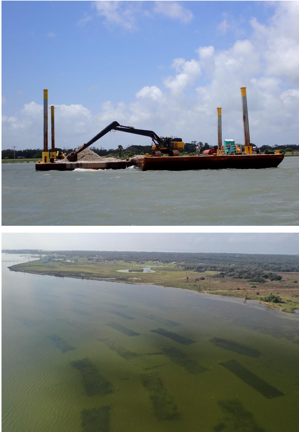
Figure 9. Restored reef construction via barge in St. Charles Bay (top) and overhead view of study area after construction (bottom, photo credit CCA Texas).
