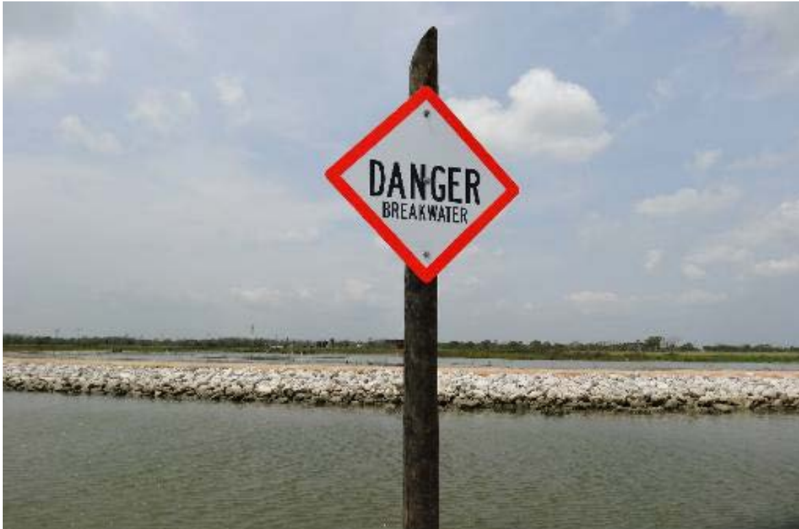
Photograph 22. Danger Signage taken east side of Marsh A.
