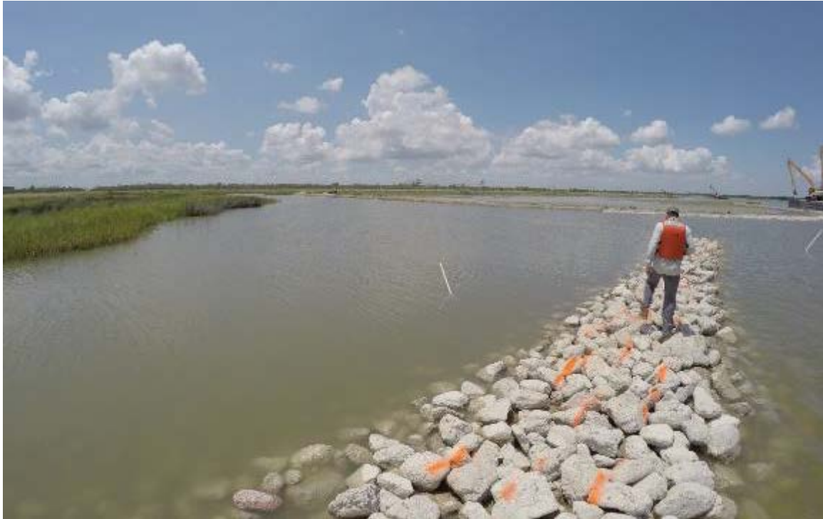
Photograph 9. Post Construction of Living Shoreline II with HDR Engineer on August 3, 2016.
