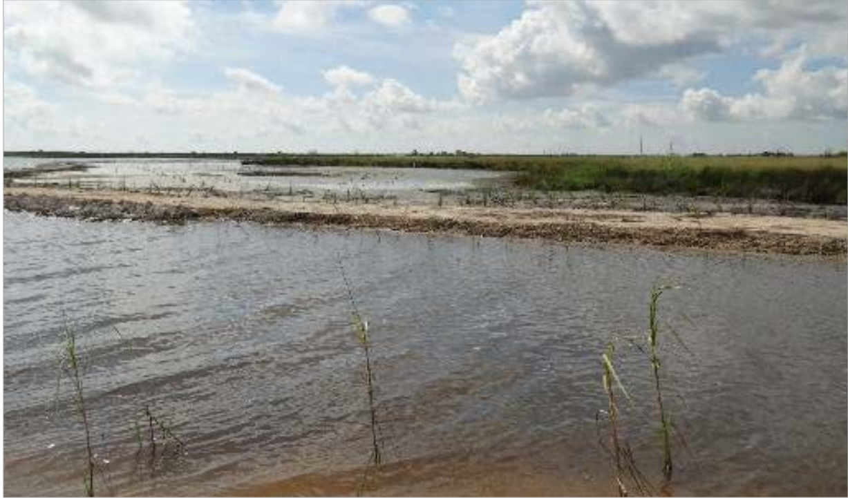
Photograph 19. Post construction planting on north side of Marsh B taken from berm on Marsh A on August 12, 2016.
