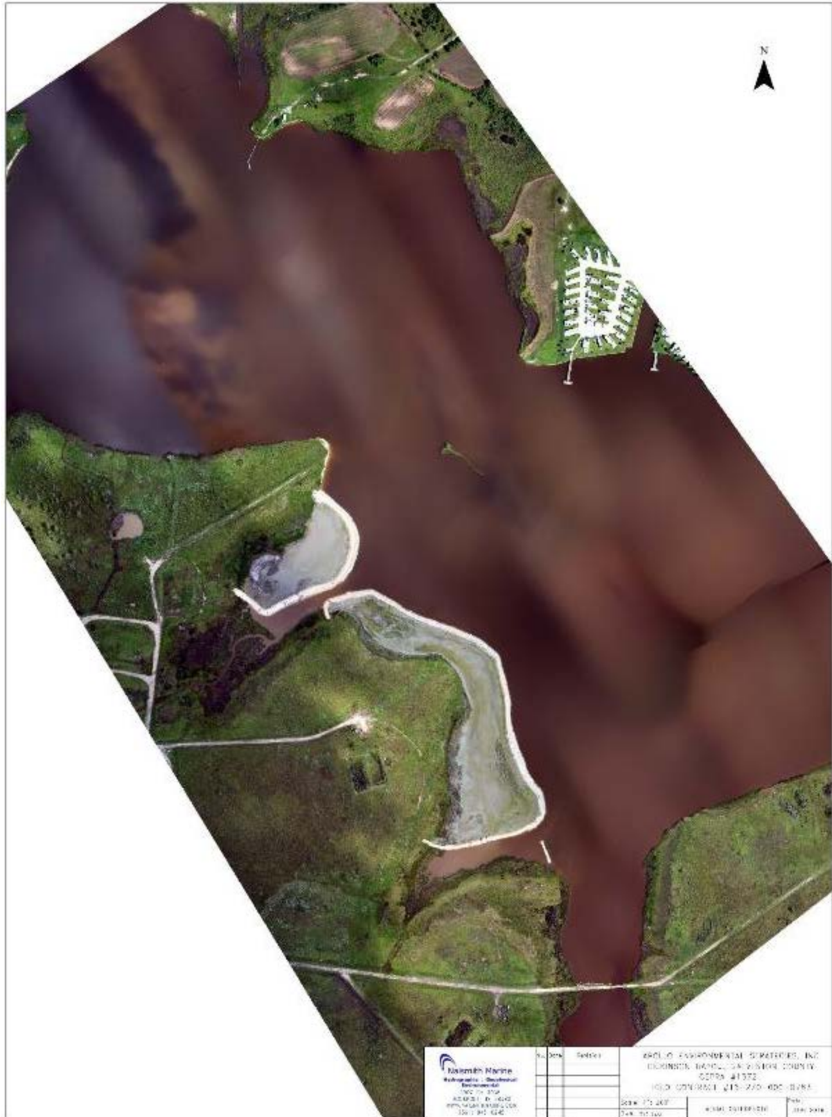
Figure 1. Final Post Construction Aerial Photograph taken by Naismith Surveying August 2016.
