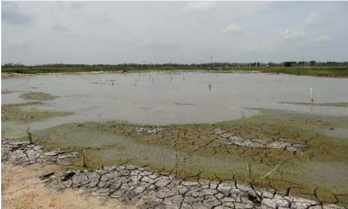
Photograph 17. Post construction planting from west side of Marsh A taken in north east direction from top of berm on August 12, 2016.
