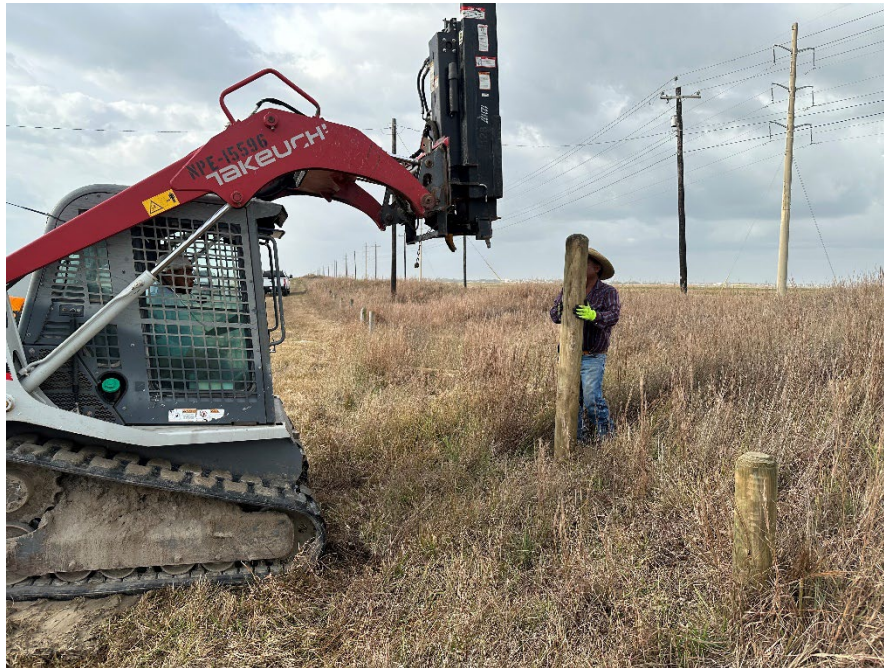
Figure 7: Installing bollards
