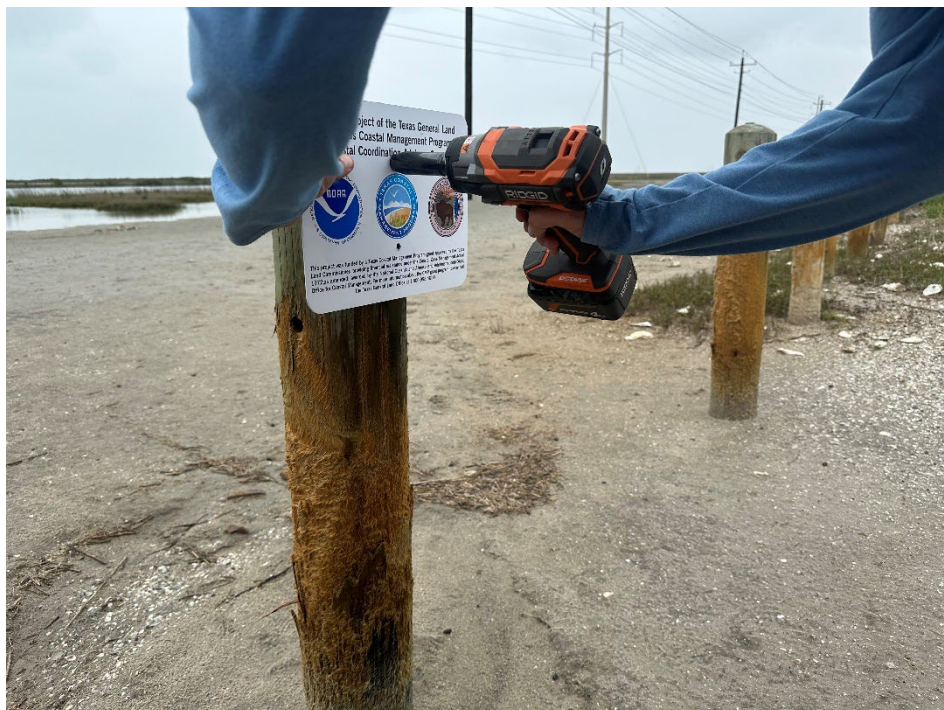
Figure 14: installing permanent CMP signage
