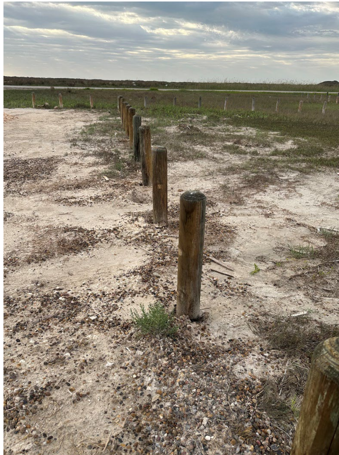
Figure 9: installed bollards around parking area
