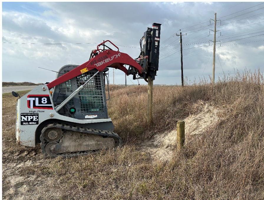
Figure 8: using hydraulic hammer to install bollards
