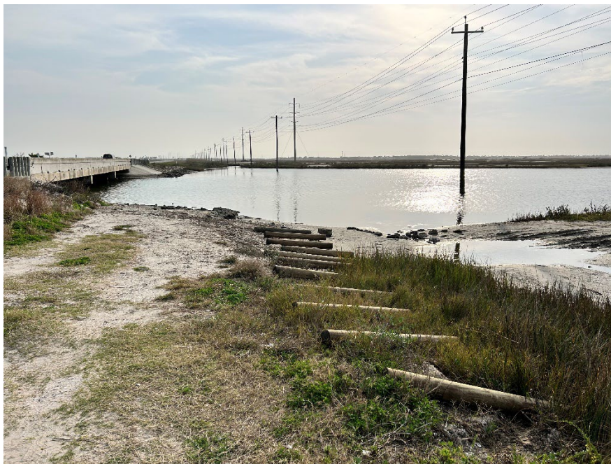
Figure 6: Bollards placed to be installed
