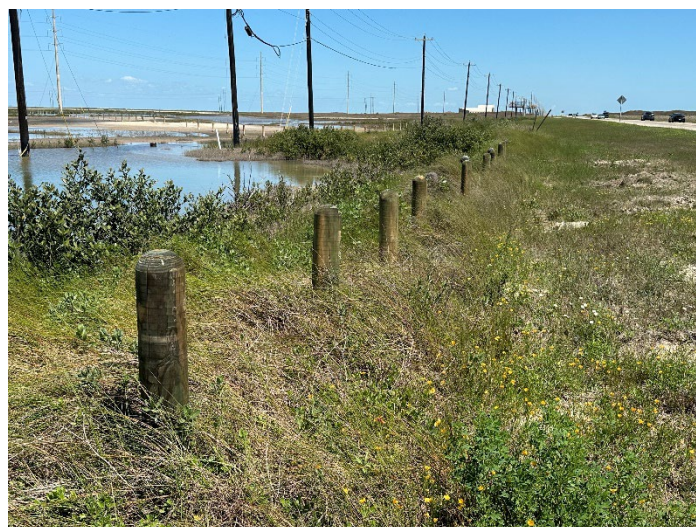
Figure 10: installed bollards along HWY 361
