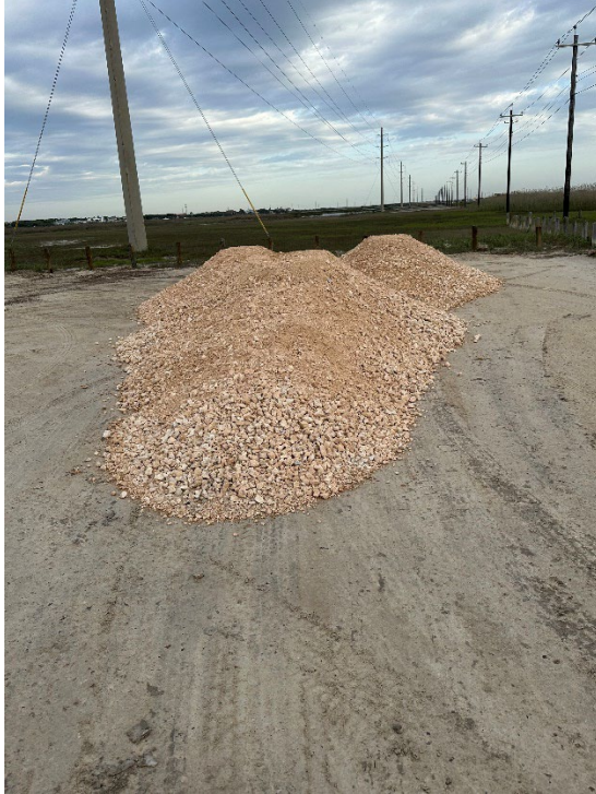
Figure 17: Spreading limestone road base
