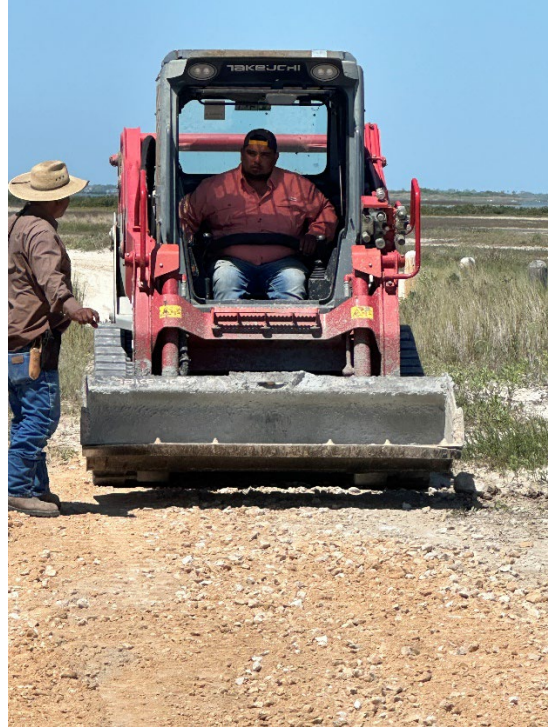
Figure 18: limestone road base
