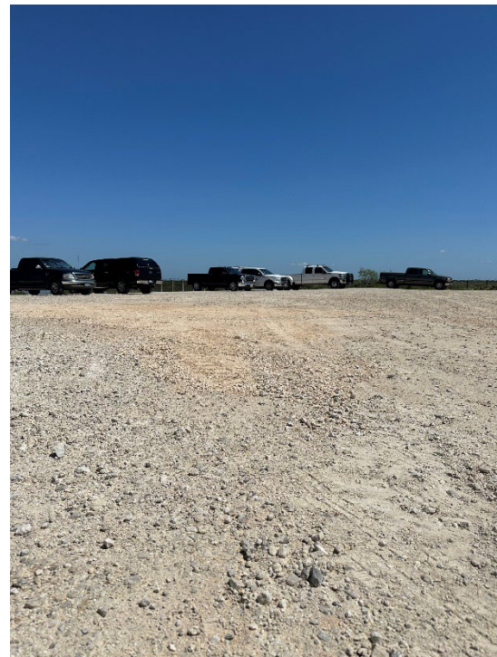
Figure 20: material added to parking area
