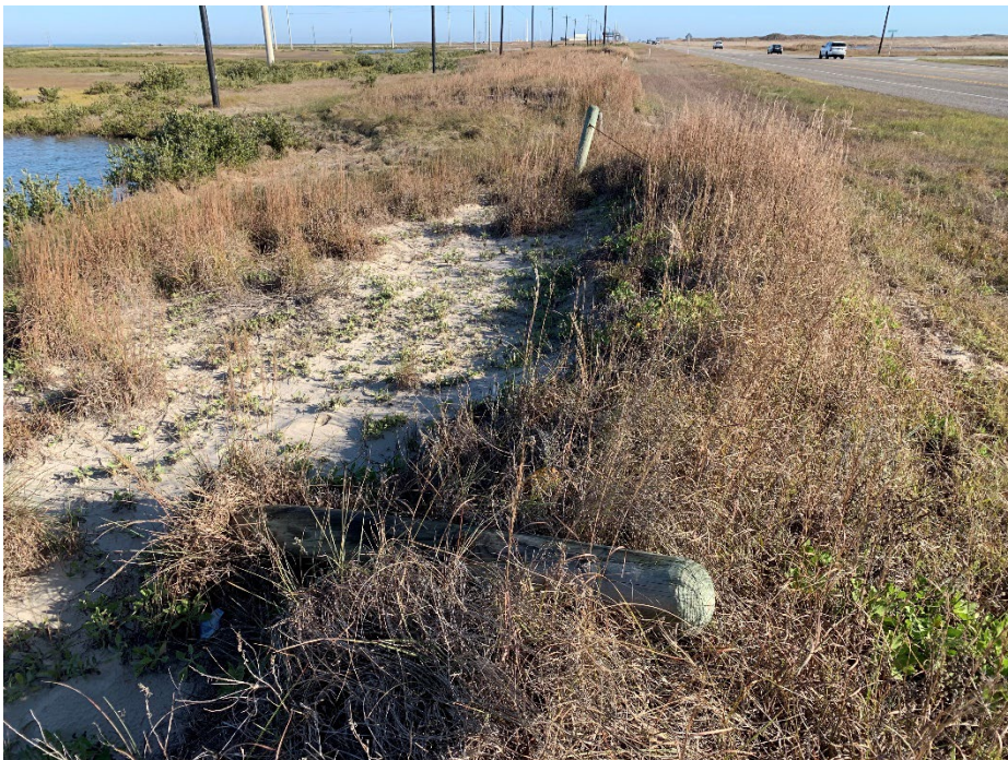
Figure 2: Example broken bollard before construction.
