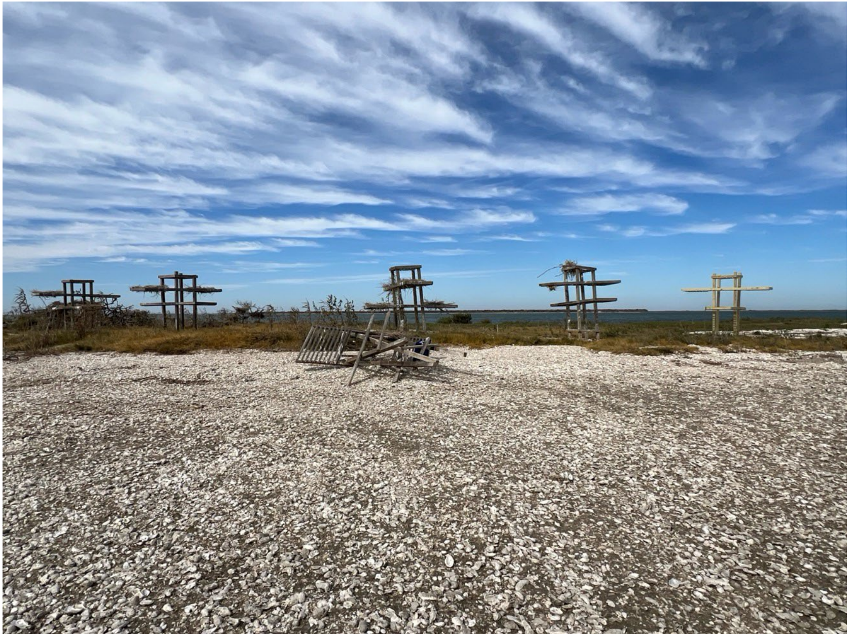
Figure 9. The largest Second Chain spoil island in February 2025 after being overwashed by tropical weather systems during the summer of 2024.
