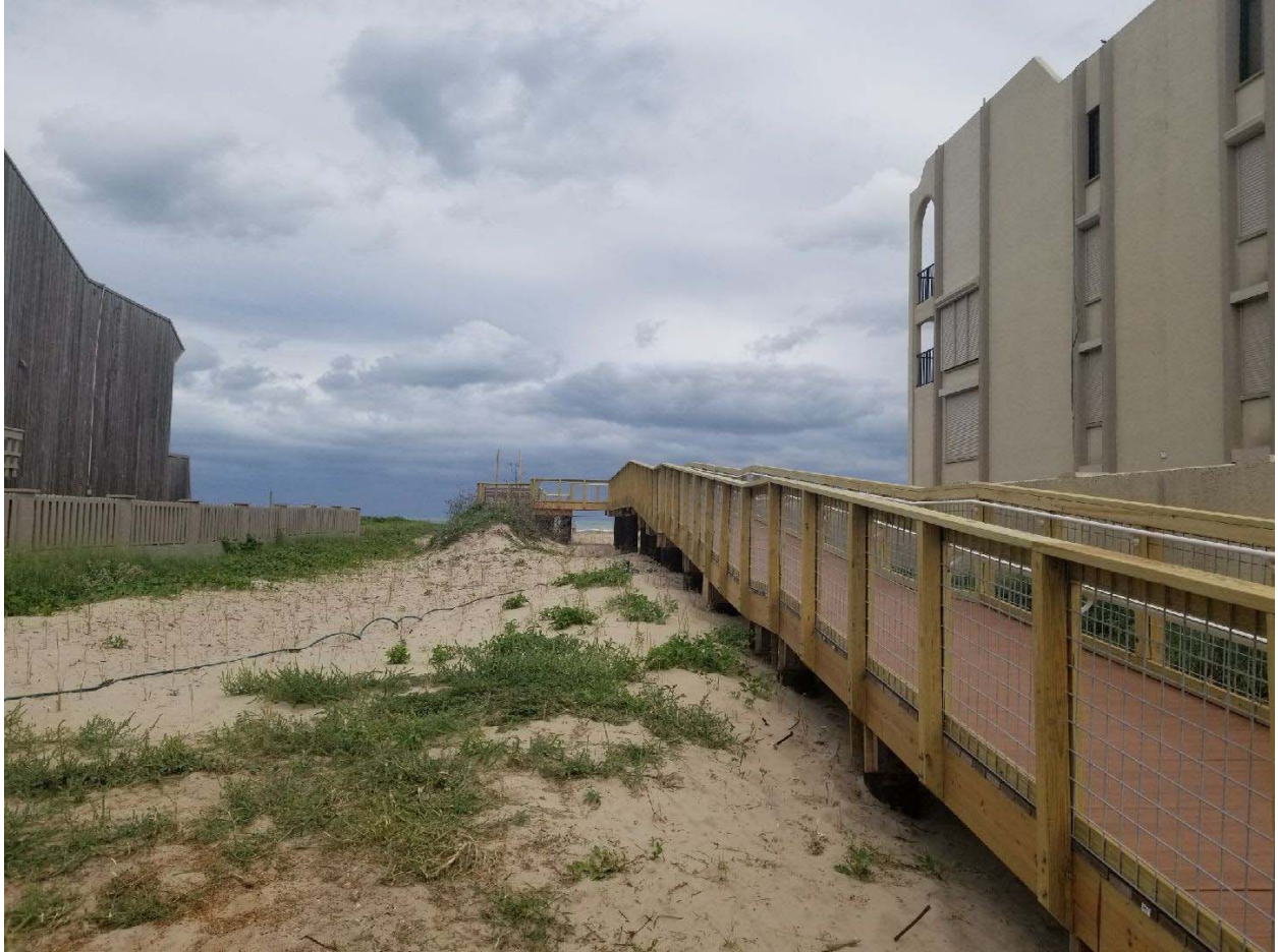
Figure 5. Photo of completed ADA-compliant dune walkover and dune mitigation post construction
