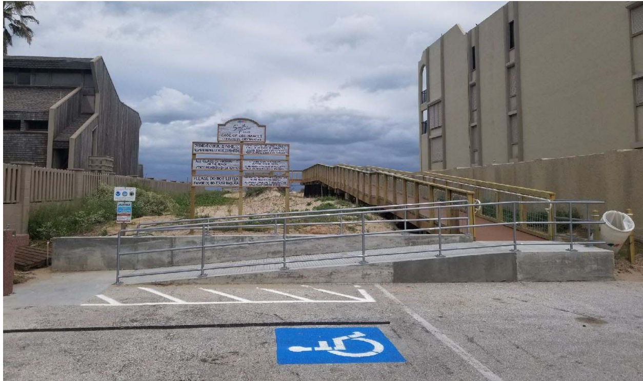
Figure 3. Photo of completed ADA-compliant dune walkover post construction
