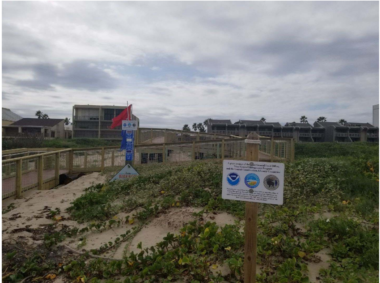
Figure 7. Photo of completed ADA-compliant dune walkover and dune mitigation post construction
