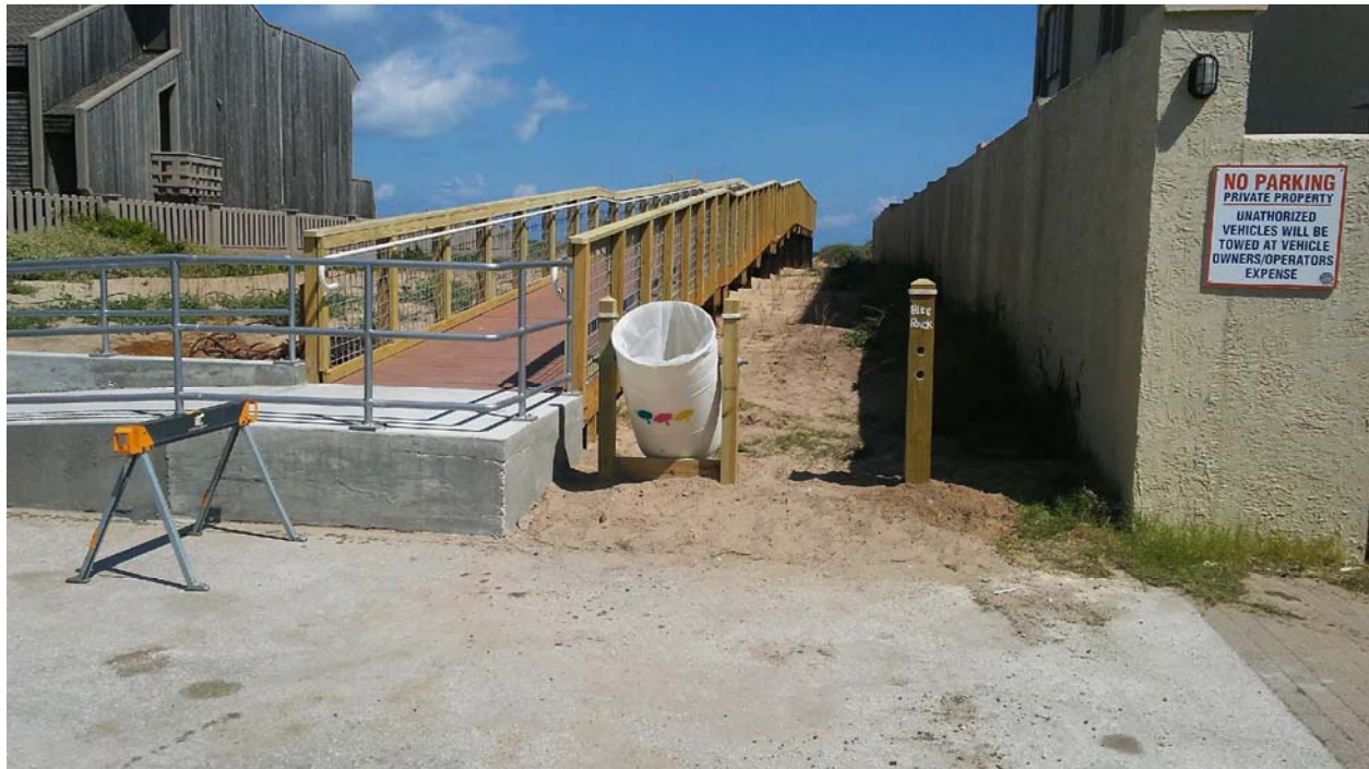
Figure 2. Photo of completed ADA-compliant dune walkover post construction
