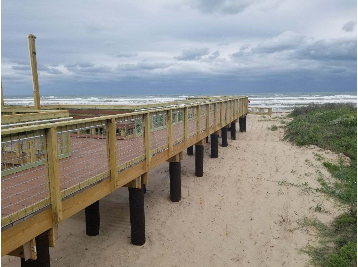
Figure 4. Photo of completed ADA-compliant dune walkover post construction
