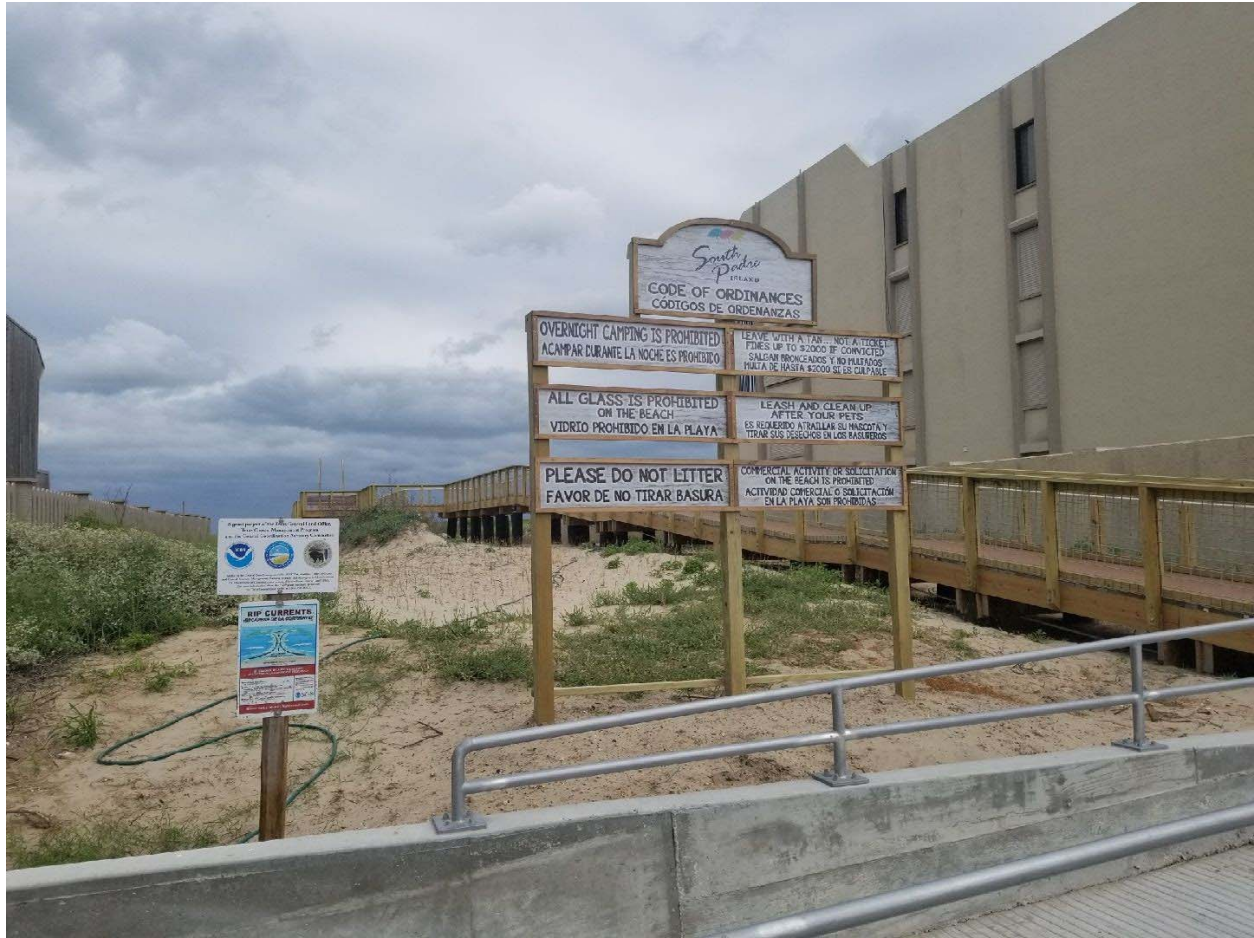
Figure 6. Photo of completed ADA-compliant dune walkover and dune mitigation post construction
