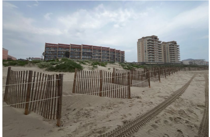
Figure 11. Discontinuous sand fencing should be no more than 10 feet long placed in segments approximately 10 feet apart, facing the predominant wind direction at a 35- to 45-degree angle to the shoreline.
