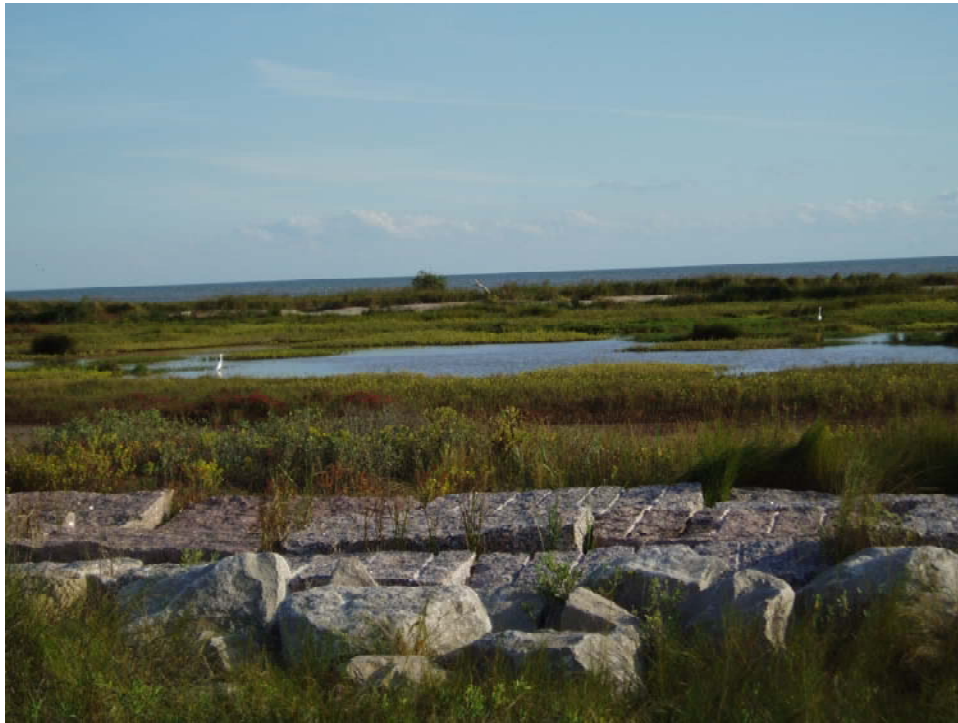
Figure 22. Top of shoreline protection feature constructed to protect the GIWW between Caney Creek and Cedar Lakes. View is gulfward.
