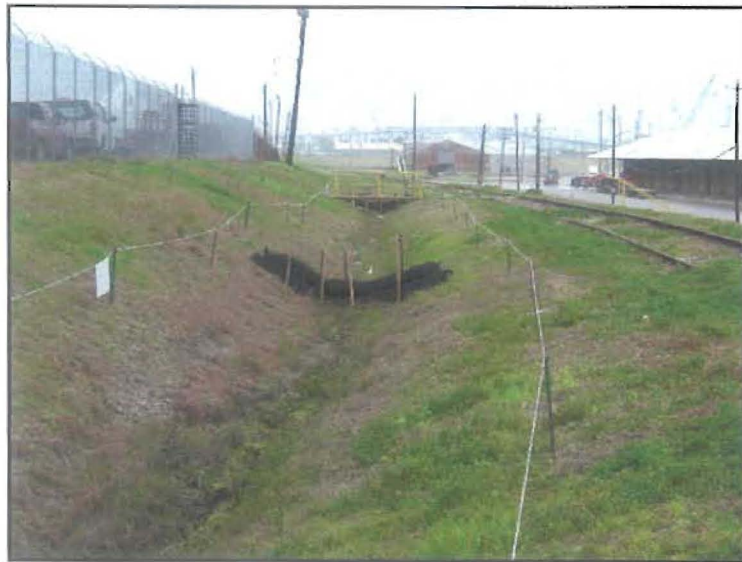
Mulch Socks and Rope Barricade
