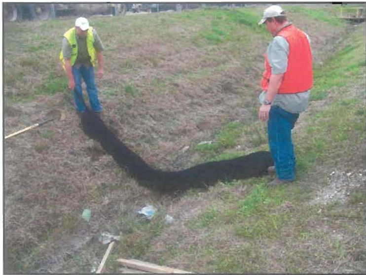
Installation of Mulch Socks
