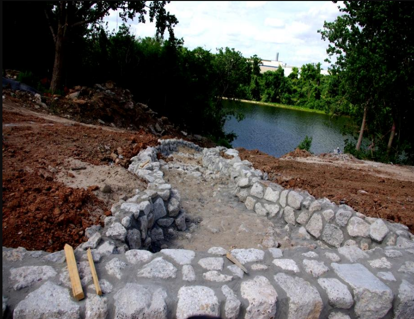
Below: spillway for carrying treated wetland overflow to the Buffalo Bayou
