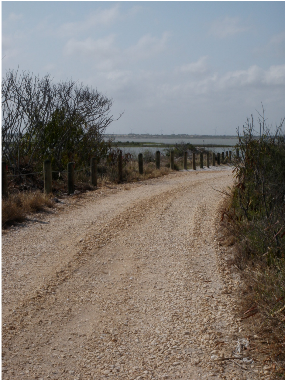
Access road to Nueces Bay Marsh Public Access Site
