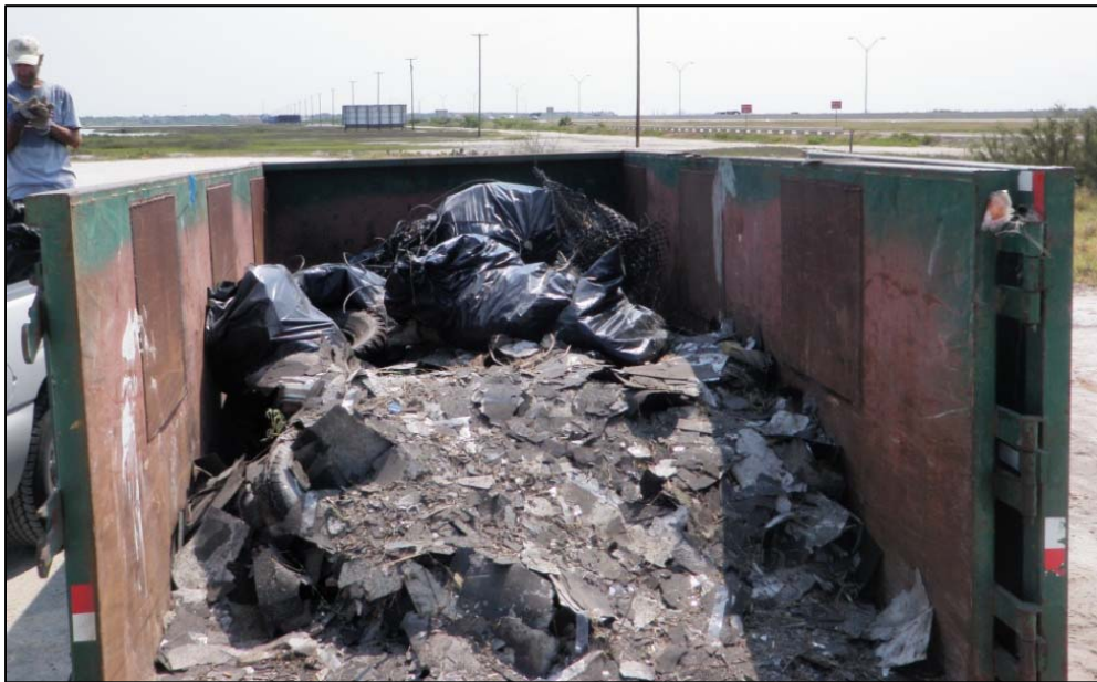
Debris removed from the access site prior to construction
