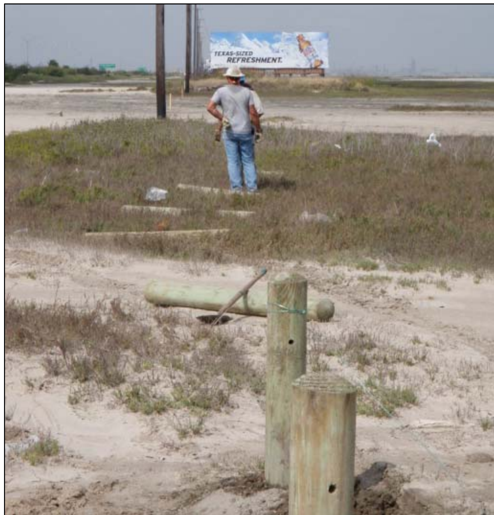
Workers installing bollards along TxDot ROW
