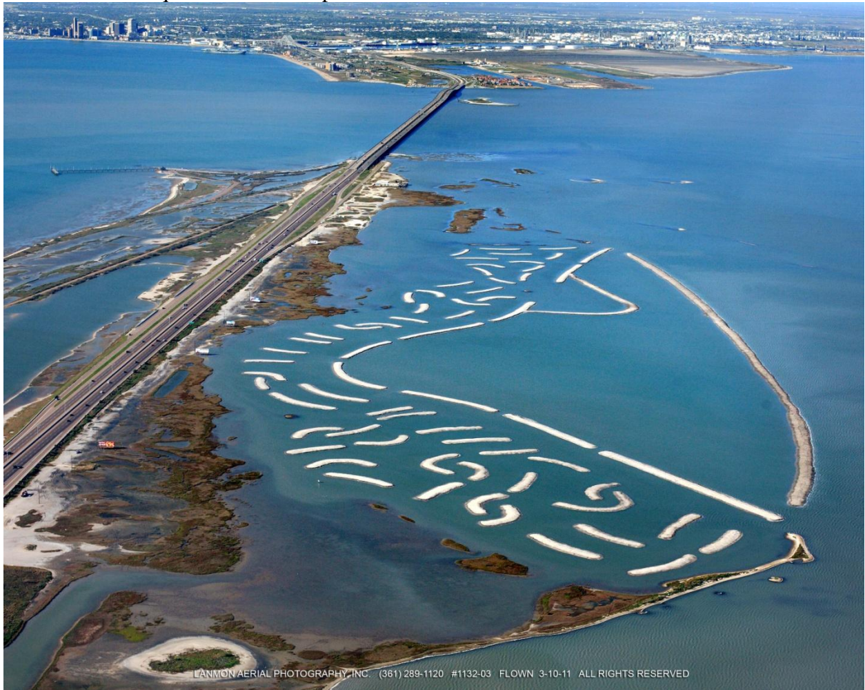
Oblique Aerial of Completed Terraces and Protective Berms: 03/06/11
