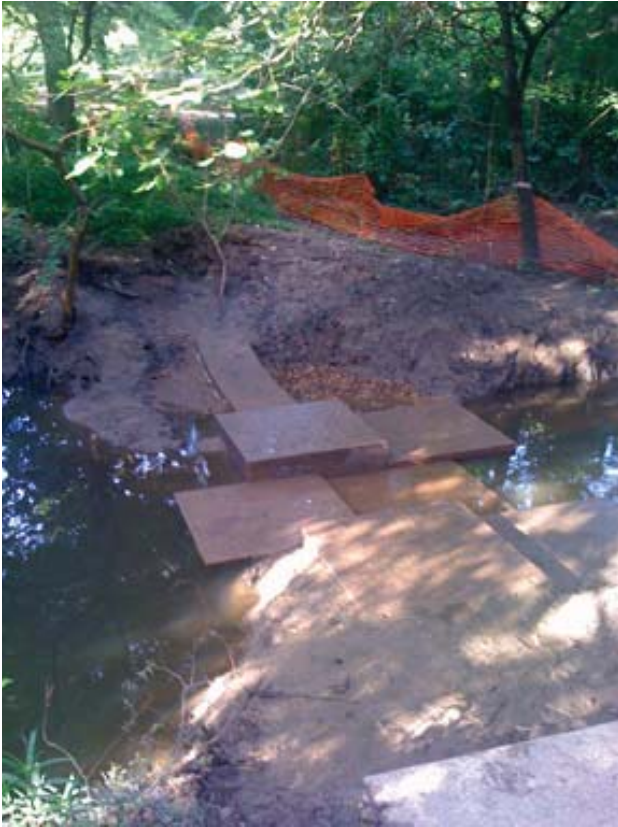
Spillway repairs at Turtle Pond . Installation of gravel fill and rubber backing.
