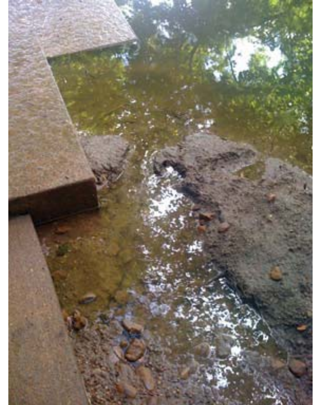
Spillway repairs at Turtle Pond . Installation of gravel fill and rubber backing.
