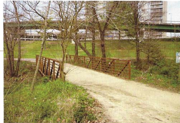
12 'Specimen Bridge at Tapley Tributary (just west of new bridge location)
