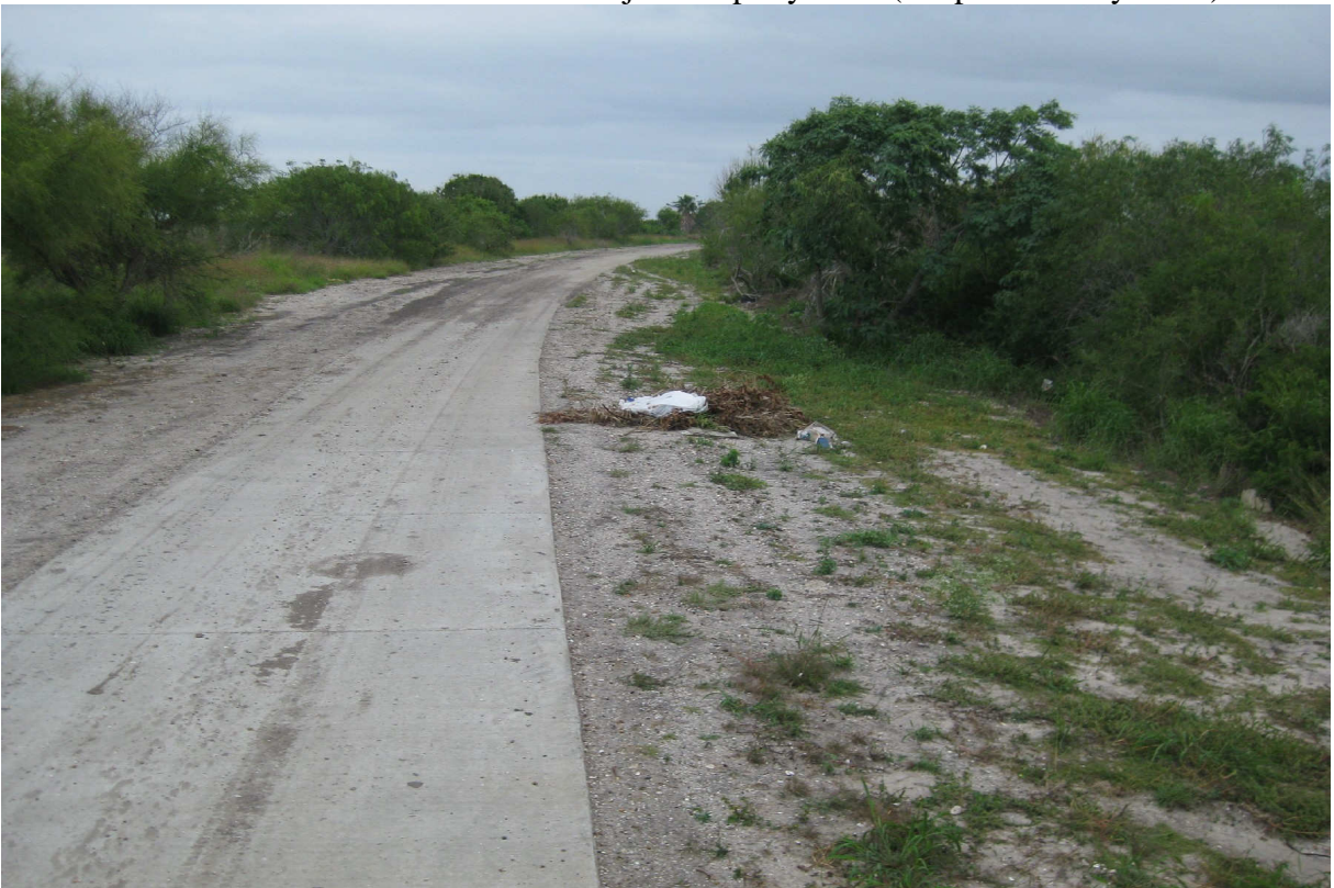
View of the North Boundary of the Subject, looking East along (unopened Holly Road). Subject is to the Right.
