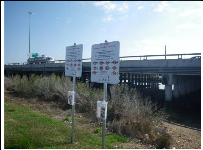
I-10 Service Road 3
