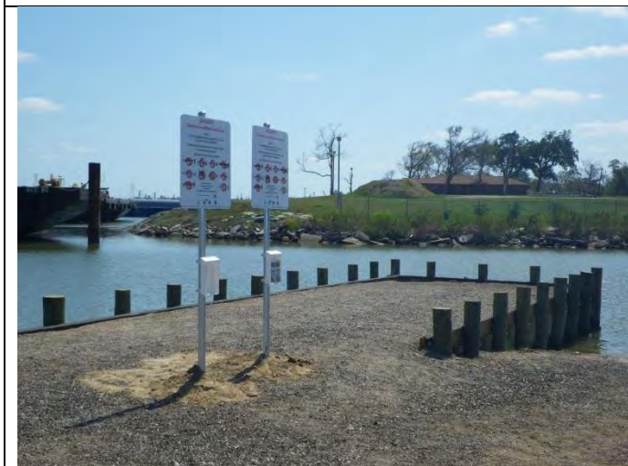
River Terrace Park Bulkhead South
