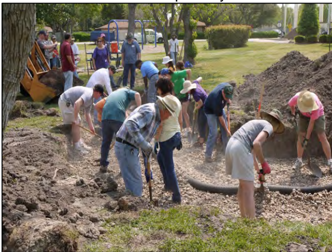
Underdrain and gravel layer installed
