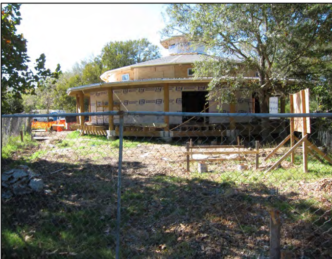
New visitor center at ABNC under construction
