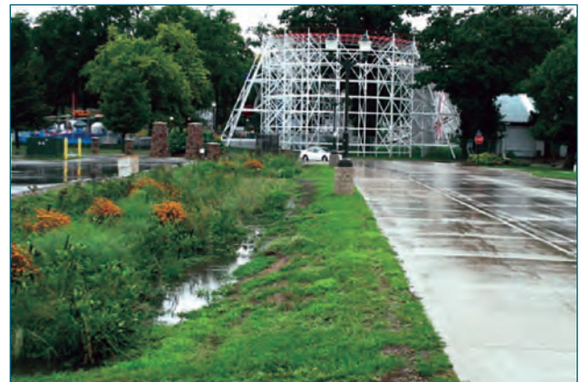
Figure 2. Rain garden built as an island in a parking lot. (Source: United States Department of Agriculture, Natural Resources Conservation Service)
