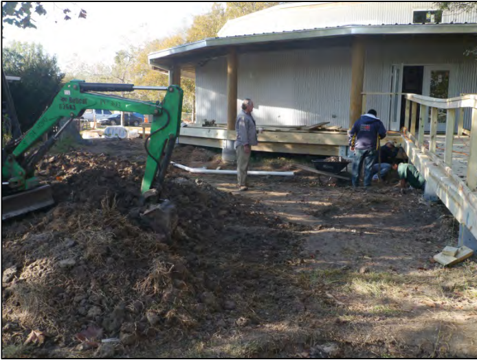
Rain garden site preparation
