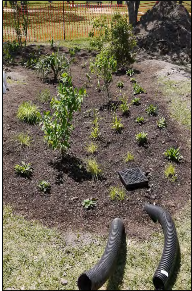
Completed rain garden showing underdrain and overflow catchment pipe
