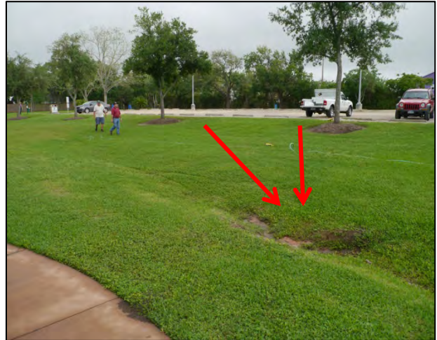
View of site from stormdrain area Arrows indicate direction of flow
