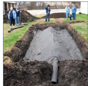
Figure 6. Placing the filter fabric.
