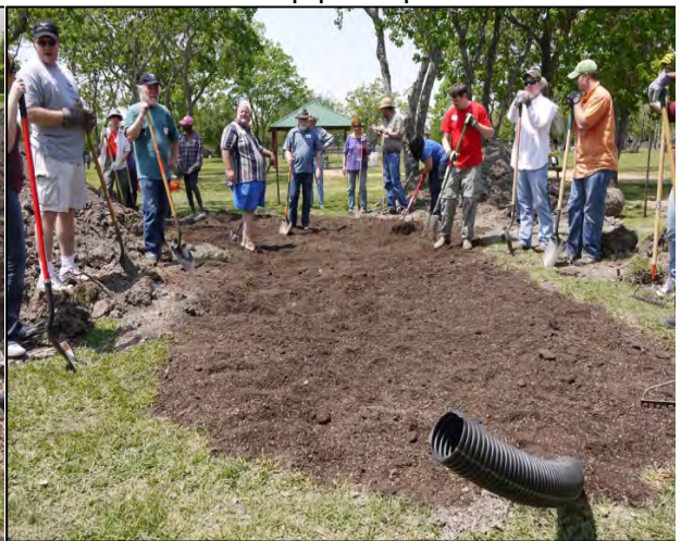
Soil in place and ready for grading
