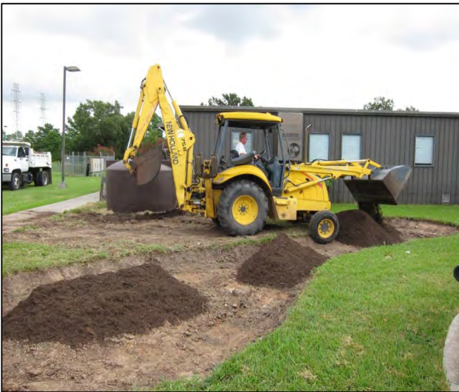
Excavation and site preparation
