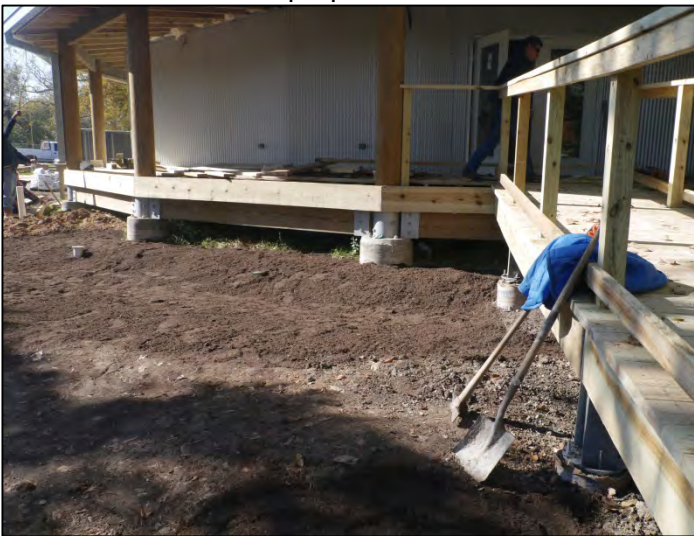
Site ready for planting
