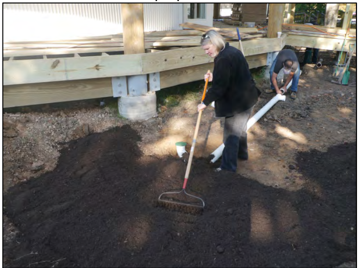
Final grading of the site
