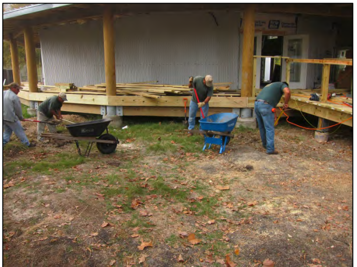
Excavating site of rain garden
