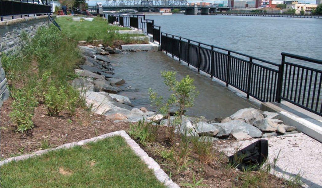
The New York Coastal Program partnered with the New York City Department of Parks & Recreation to construct a portion of Harlem River Park, part of the Manhattan Waterfront Greenway. The project used an innovative design approach that incorporated durable, textured materials to absorb wave/wake energy and mitigate storm surge, staggered gabions seeded with oyster shells to foster habitat and enhance water quality, a kayak launch, and a constructed tide pool (pictured above at high tide). Credit: NYDOS
