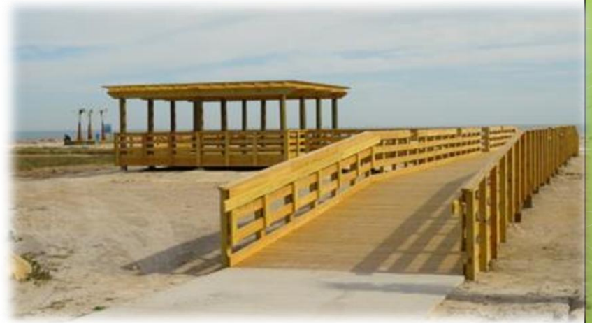
View of ramp and covered area facing South
