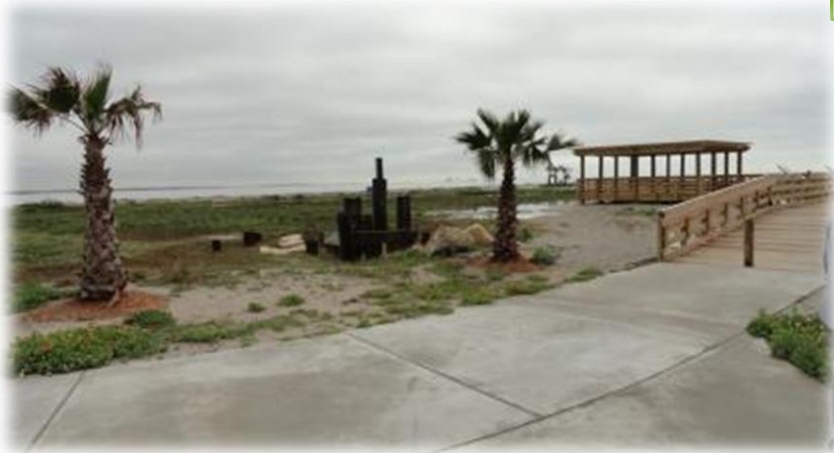
Beachwalk new GLO sign location
