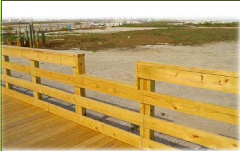
Promenade prior to signage installation
