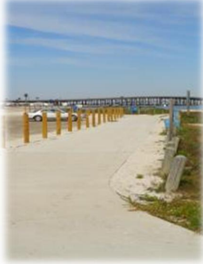
Sidewalk north towards the Harbor Bridge
