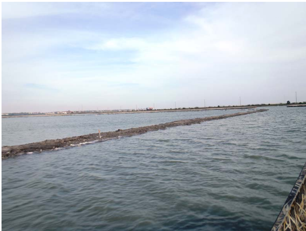
Cell 3 Toe Berm.
