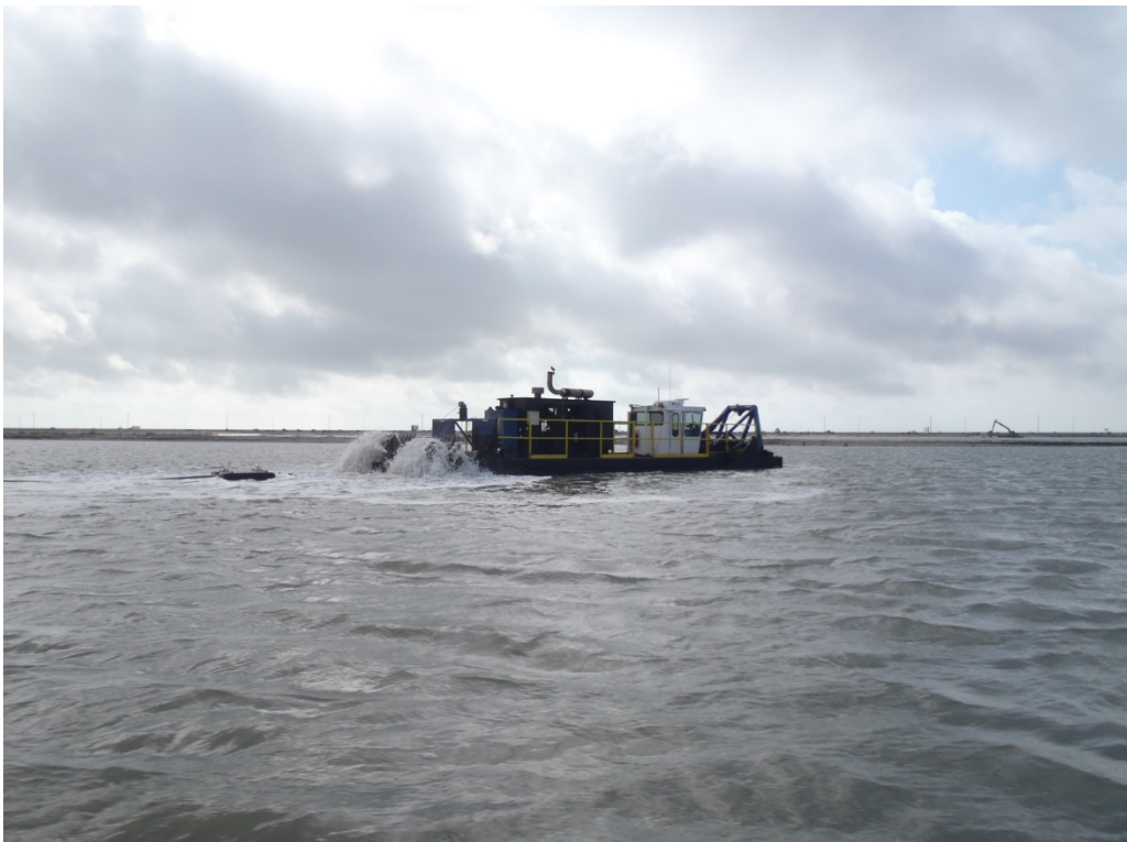
Ike dredging within Borrow Area A.
