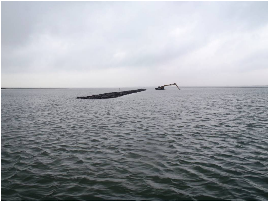
Construction of Cell 3 Toe Berm.
