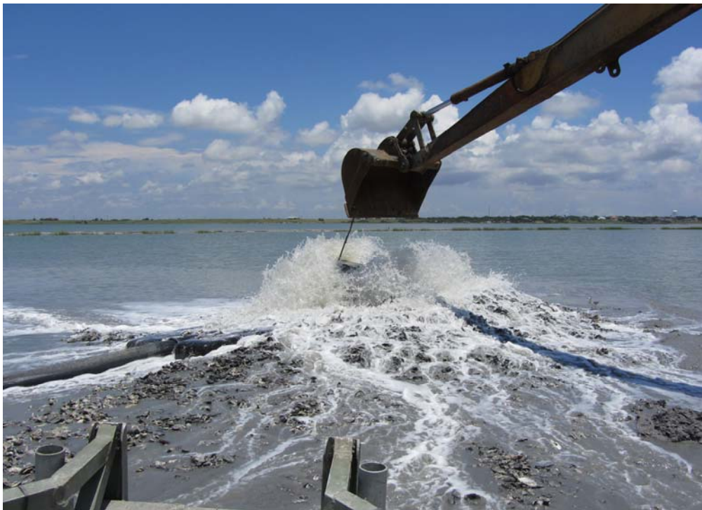
Construction of marsh mound M7.
