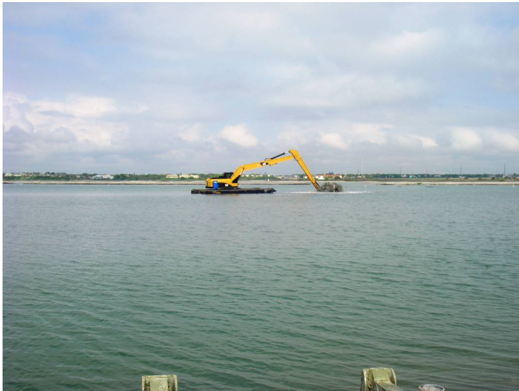
Marsh excavator securing dredge pipe at M11 discharge point.
