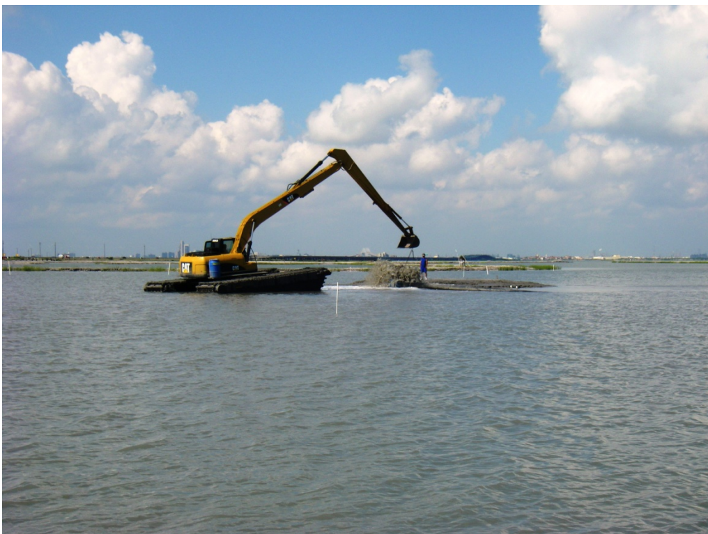
Dredge discharging at marsh mound M1.
