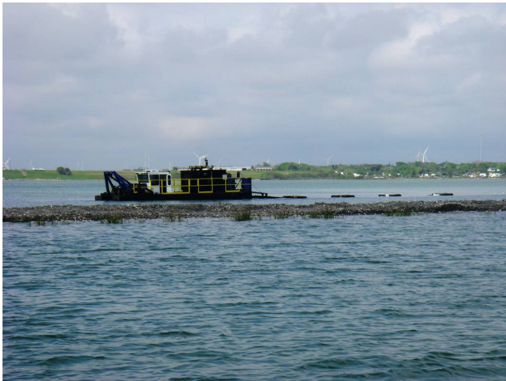
Ike dredging within Flotation Channel/Borrow Area A.
