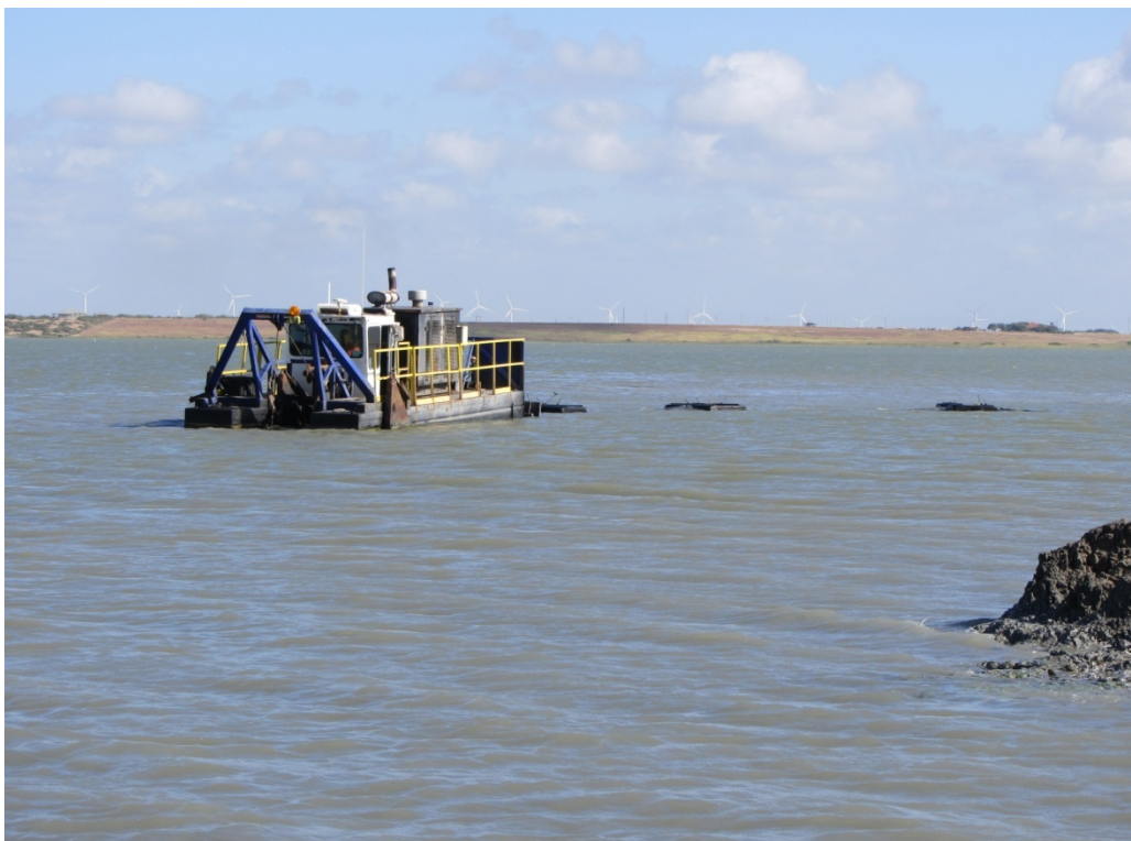
Dredge located near the end of Reach 1.
