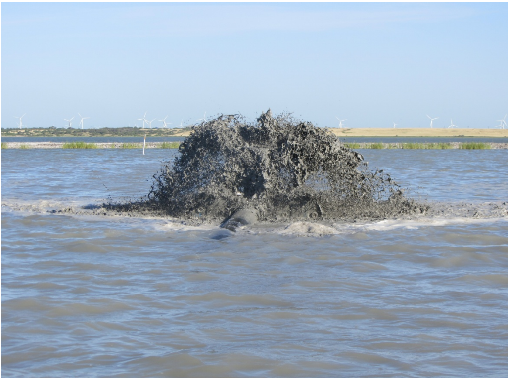
Dredge discharging at marsh mound M3.
