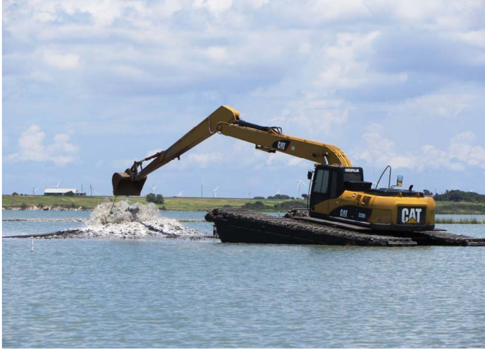
Construction of marsh mound M7.
