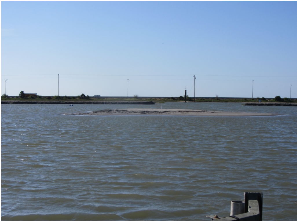
Marsh mound M11. Note equilibration of side slopes.
