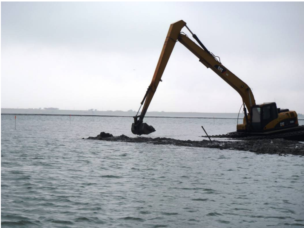
Construction of Cell 3 Toe Berm.
