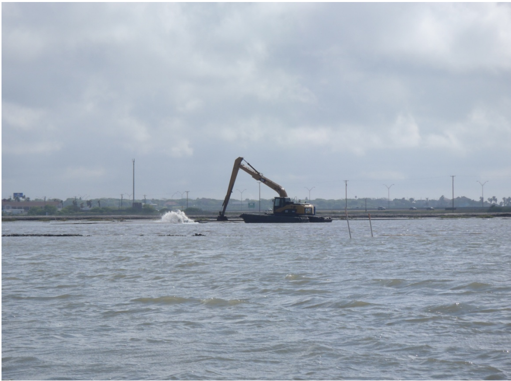
Construction of Marsh Mound M10.
