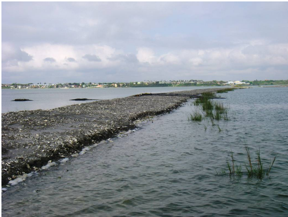
HDPE dredge pipe across outer berm.
