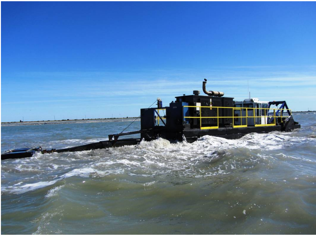
Ike dredging within Borrow Area A.
