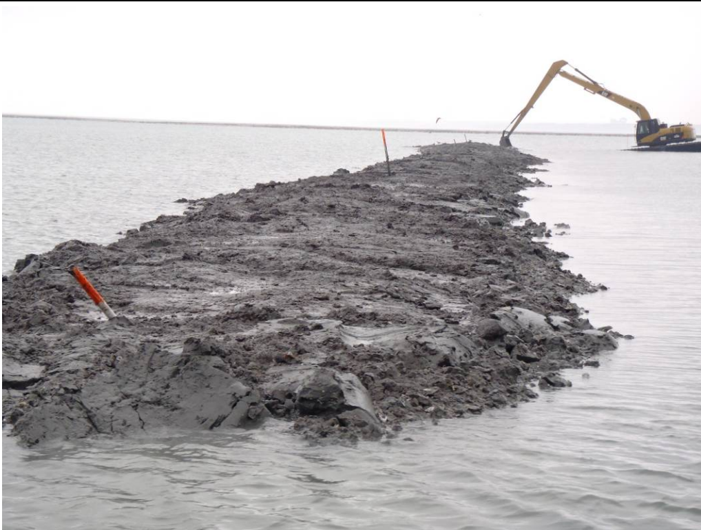
Construction of Cell 3 Toe Berm.
