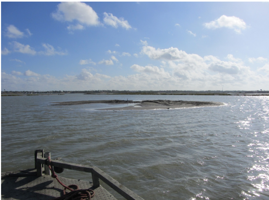
Marsh mound M8. Crest needs to be rebuilt
