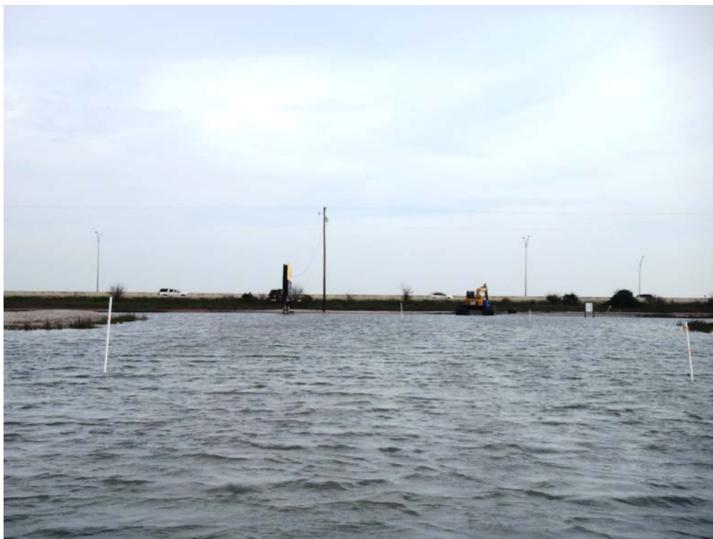
Temporary access corridor..
