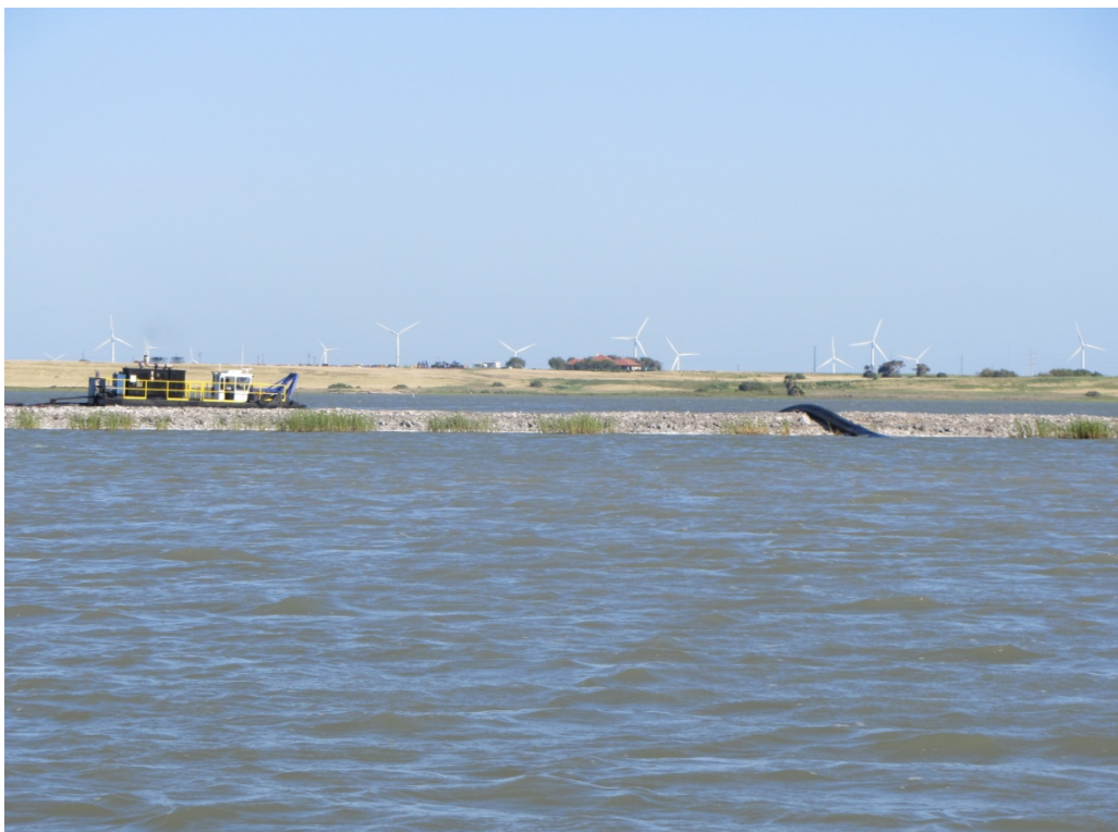
Dredge and discharge pipe over outer berm.
