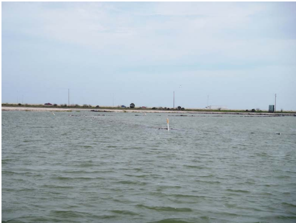
Cell 3 Toe Berm.
