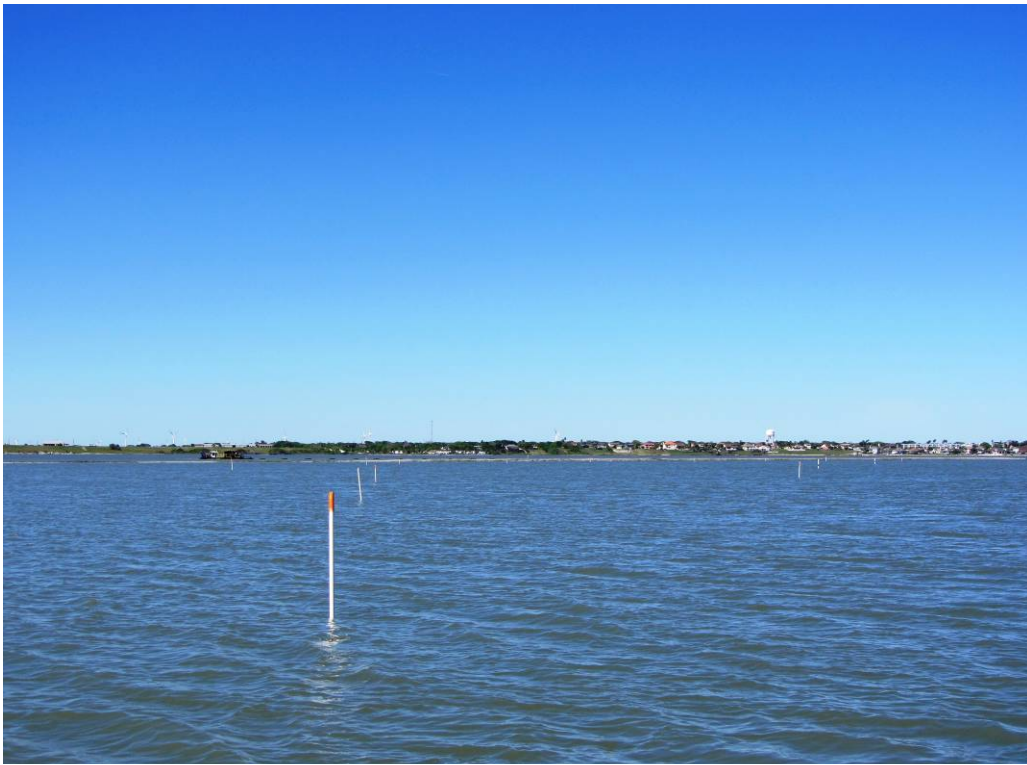
Toe berm and mound stakes.
