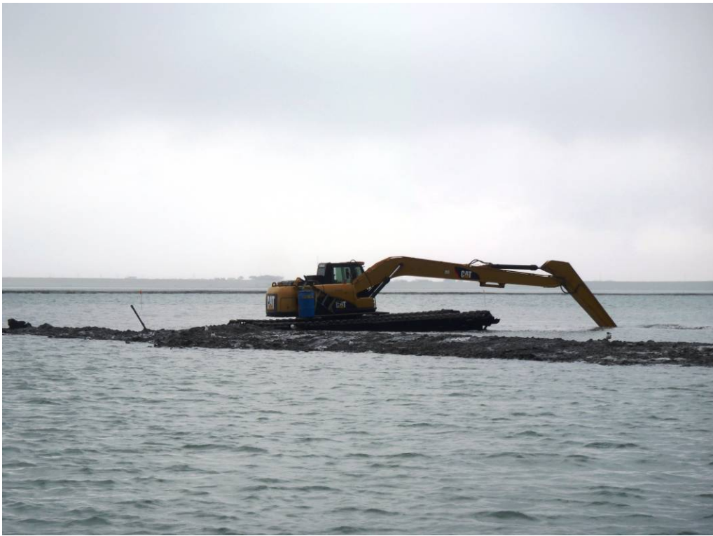
Construction of Cell 3 Toe Berm.
