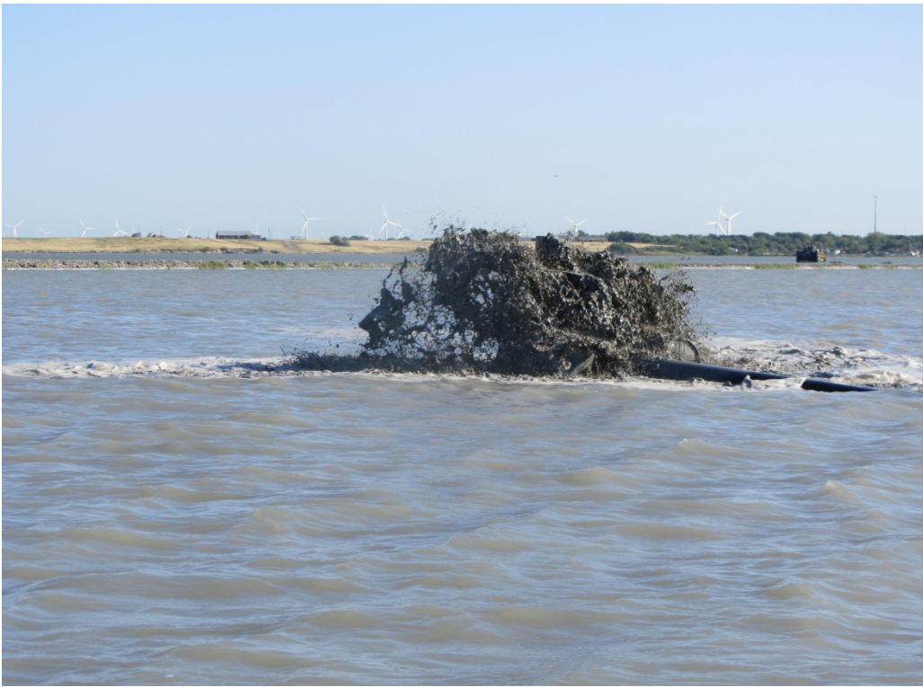
Dredge discharging at marsh mound M3.
