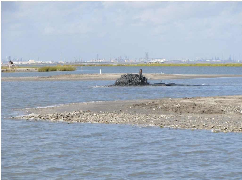
Material being pumped between M1 and M2.
