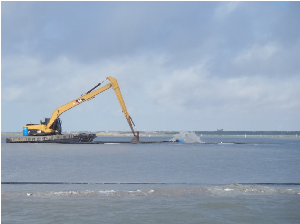
Construction of Marsh Mound M10.
