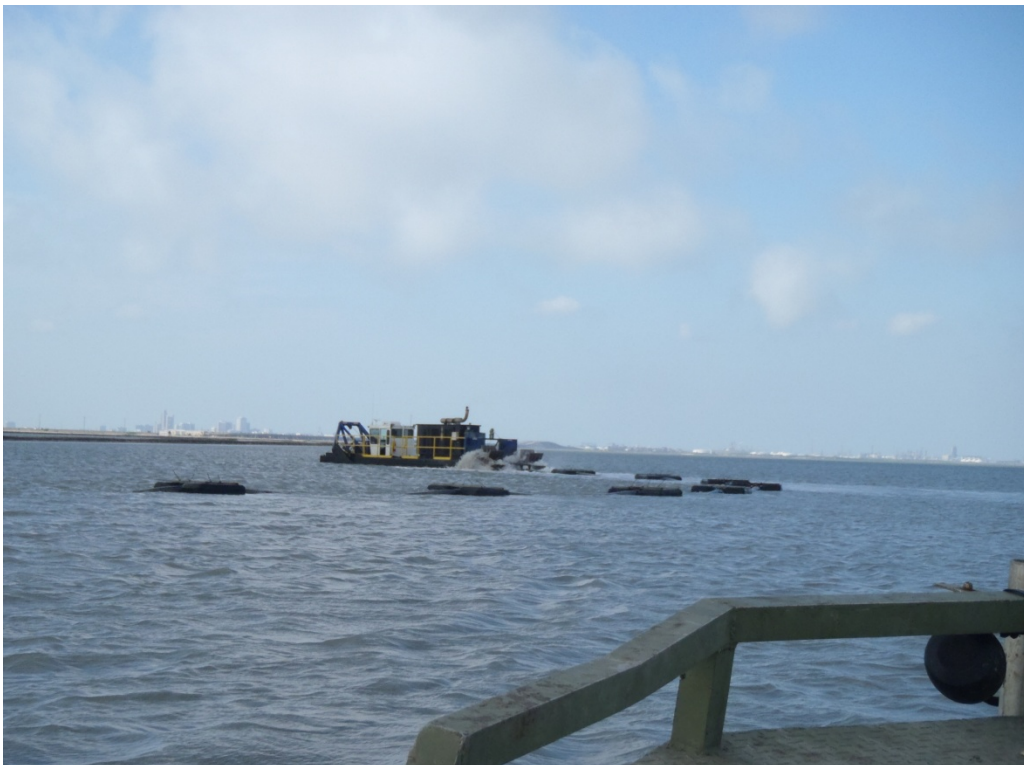
Ike dredging within Borrow Area A.
