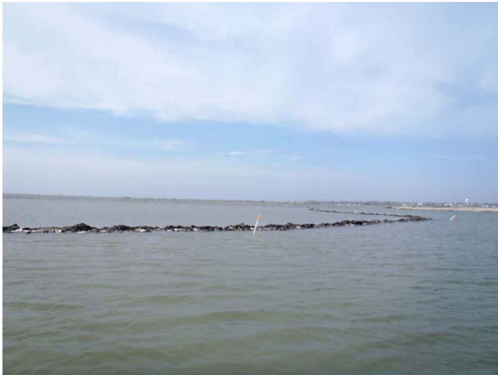
Cell 3 Toe Berm.
