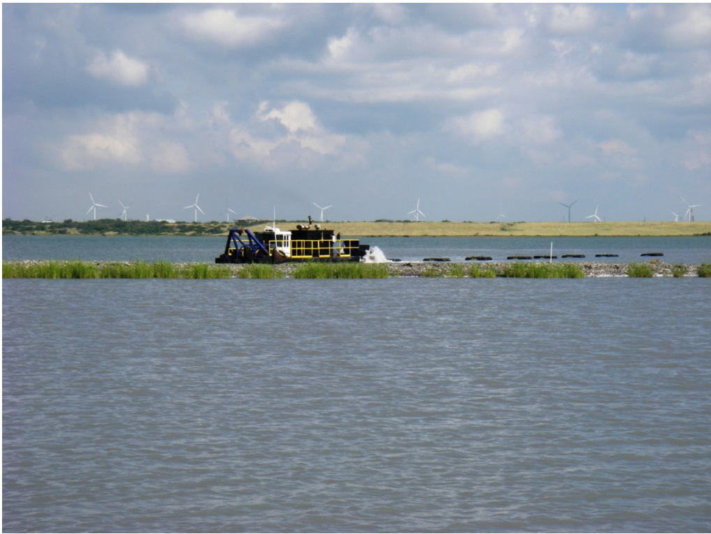
Ike dredging within Borrow Area A.
