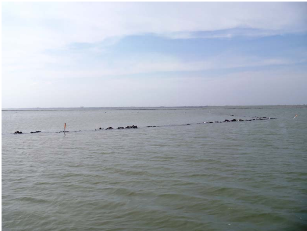
Cell 3 Toe Berm.
