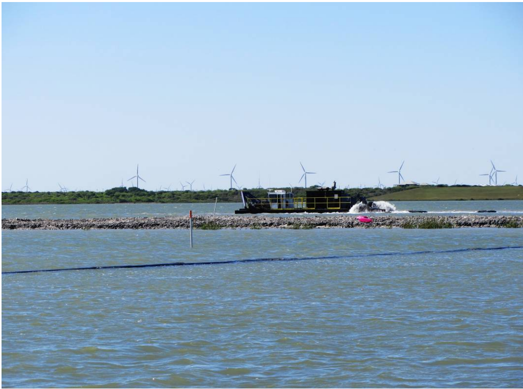
Ike dredging within Borrow Area A.
