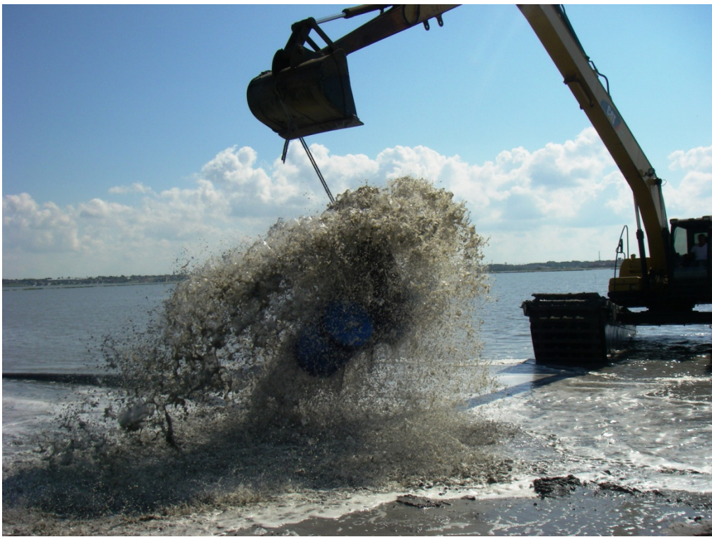
Relocating dredge pipe at marsh mound M1.
