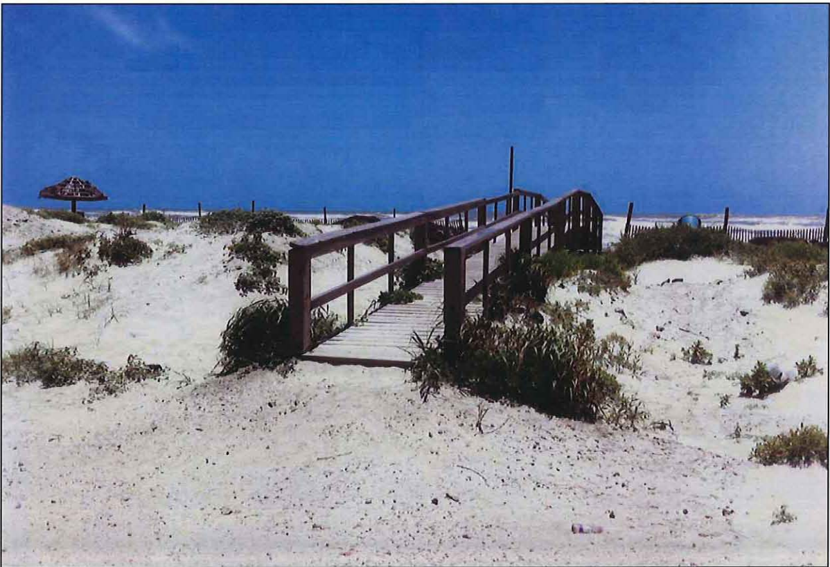
N. Village of Surfside Beach: Pedestrian Beach Access Point at Sand Dune Ct. (IMG_0670.JPG)
