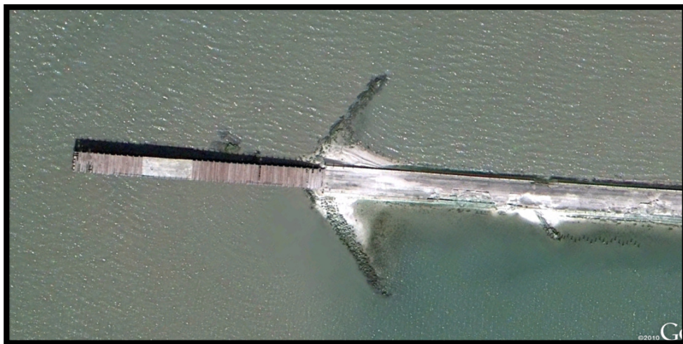
Abandoned Fishing Pier
