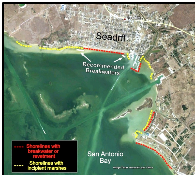
Figure B7. General physical characteristics of the shorelines at Seadrift, showing areas that have hard structures, areas with incipient marshes, and recommended areas for breakwaters.
