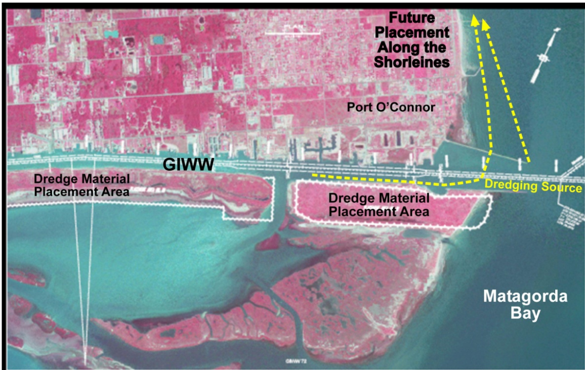
Figure B10. Dredging source for the sediments at the GIWW near Port O'Connor that are placed at the King Fisher Park. Source: Image modified from the GIWW USACE O&M Project Map Book, Galveston District.
