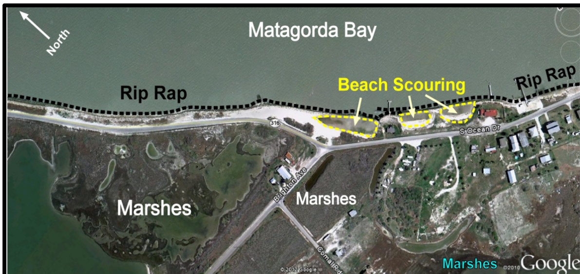
Figure B15. Distribution of concrete riprap between Magnolia and Indianola beaches. Erosion is creating a beach-scouring process behind the riprap, making the area more susceptible to environmental damage and impacts to the marshes behind these barriers.
