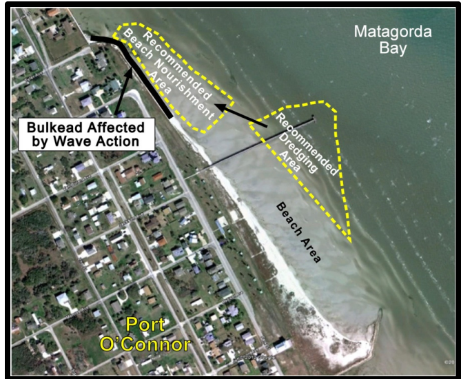
Figure B12. Potential dredging at the King Fisher Park may allow for more depth at the end of the fishing pier. The dredged sediments may be placed on the north side of the bulkhead, thereby reducing the shoreline erosion problems.
