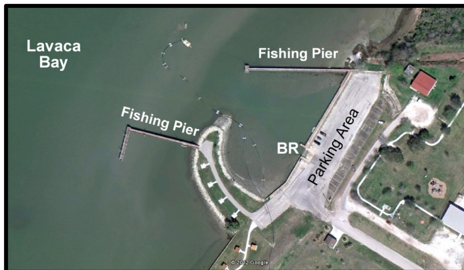
Figure 54. Point Comfort Park fishing piers.
