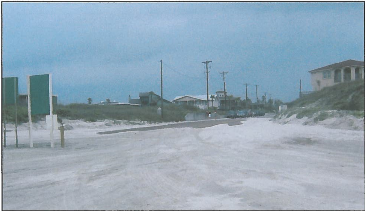
Vehicle Beach Access Point at Avenue G
