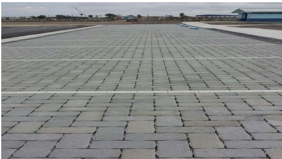
Figure 5.4. Cameron County Drainage District #1 Parking lot
