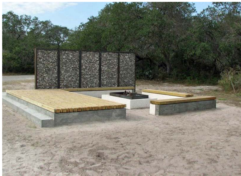
Figure 15. Shellcrete structure created from recycled oyster shells at Goose Island State Park.
