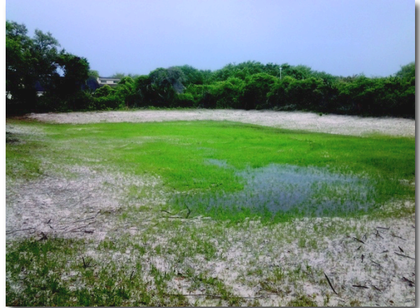
Small pond after construction.
