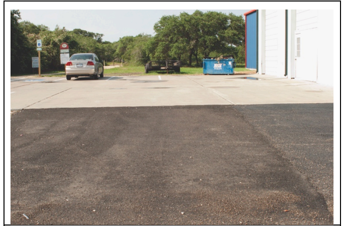
Paved section between concrete parking and street.
