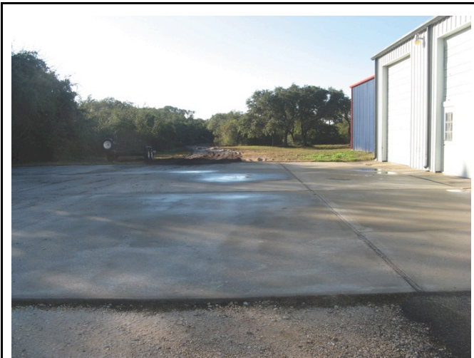
Palmetto Avenue, northeast entrance parking before construction.
