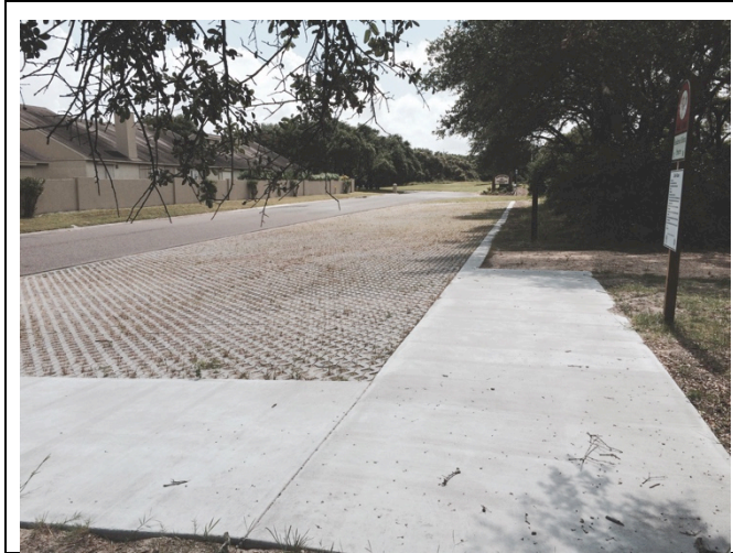
Henderson Street parking permeable parking after construction.
