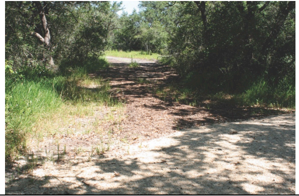
Primitive trail 1 after construction.
