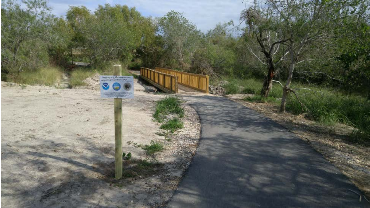
Figure 1. Photo of constructed trail, timber walkway, and installed CMP signage.
