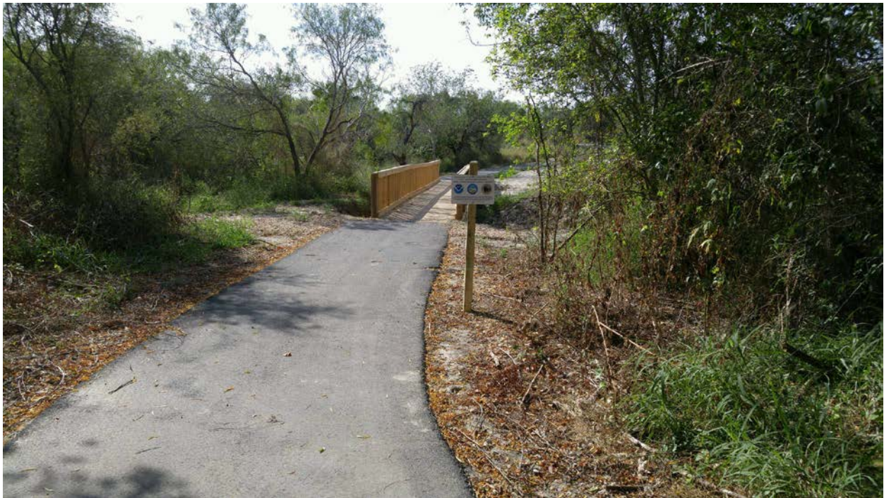
Figure 2. Photo of constructed trail, timber walkway, and installed CMP signage.
