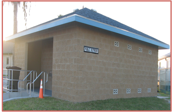
Photo 8. Post Construction East Side
