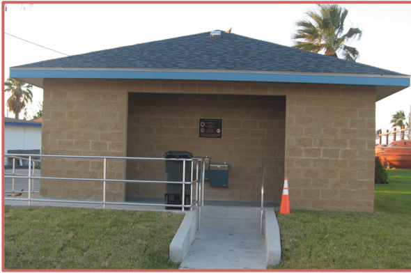
Photo 7. Post Construction Front
