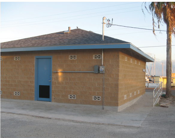
Photo 9. Post Construction Rear
